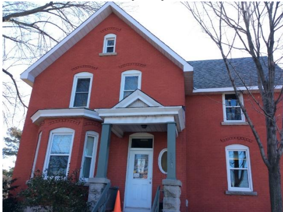
Front façade, Source: City of Ottawa, 2018
