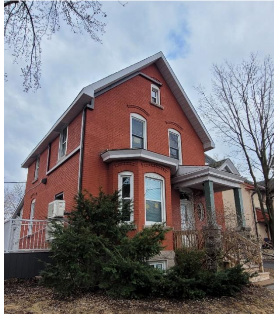
224 McArthur Avenue, northeast corner, Source: City of Ottawa, 2024
