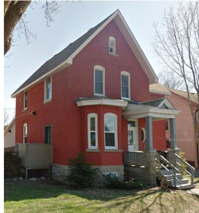
Front and east façade, Source: GoogleMaps, 2016
