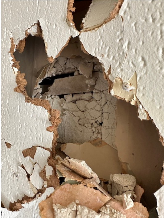
Photo 5 – Plaster Degradation (227/229)
