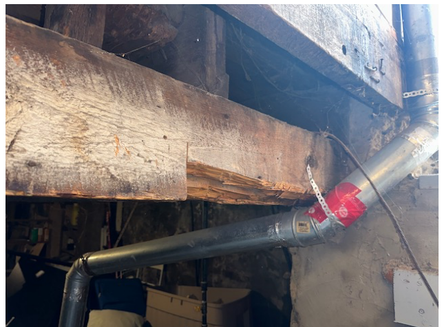
Photo 12 – Notched Joists (235/237)
