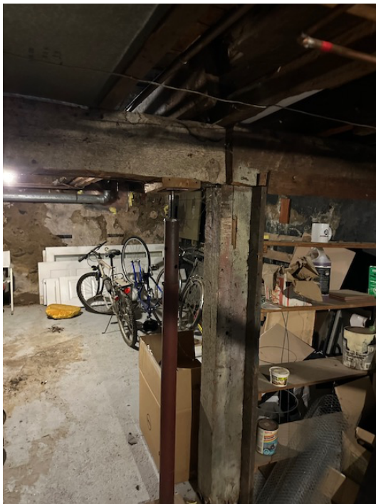
Photo 11 - Basement Framing Reinforcing (235/237)
