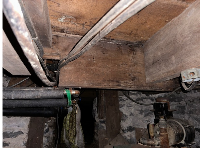
Photo 2 – Unsupported/Notched Joist (227/229)
