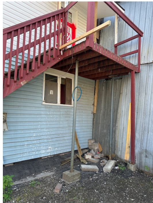
Photo 8 – Rear Elevated Deck (231/233)
