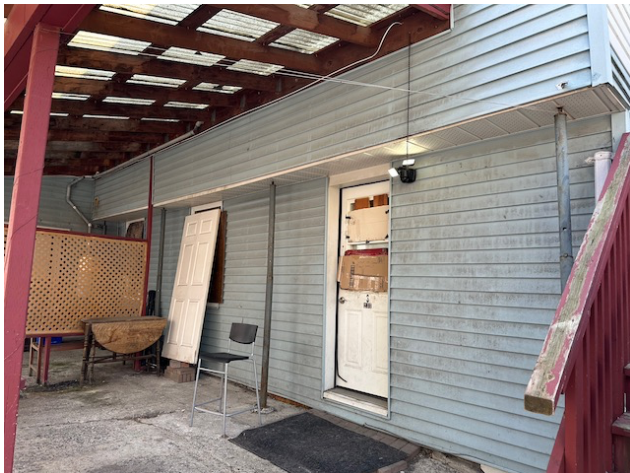
Photo 7 – Added Teleposts @ Overhang (231/233)
