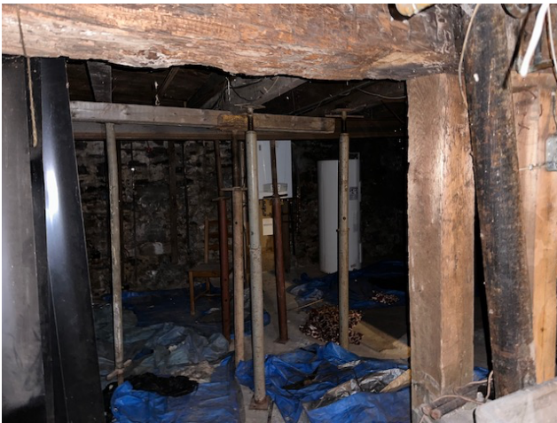
Photo 3 – Added Teleposts (227/229)
