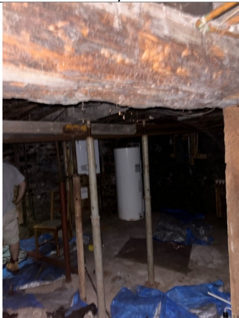
Photo 12: Temporary jackposts installed to support sagging floors.
