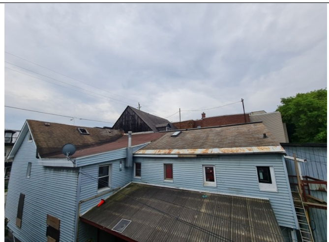
Photo 7: 231/233 St. Patrick St roof condition.
