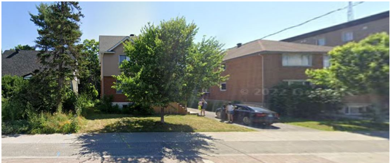
Figure 3 Subject Property Existing Condition.
