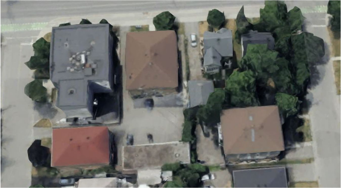
Figure 4 Subject Property Existing Rear-Yard Condition.
