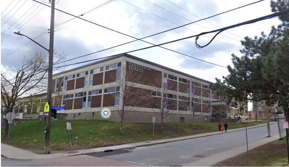
Centennial Public School. S-W corner of Bay & Gloucester.
