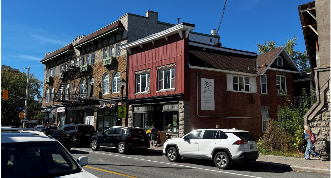
1121 Wellington Street West, adjacent to the Iona Mansions at 1123-1131 Wellington Street West (City of Ottawa)
