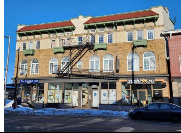
1123-1131 Wellington Street West (Image, City of Ottawa)
