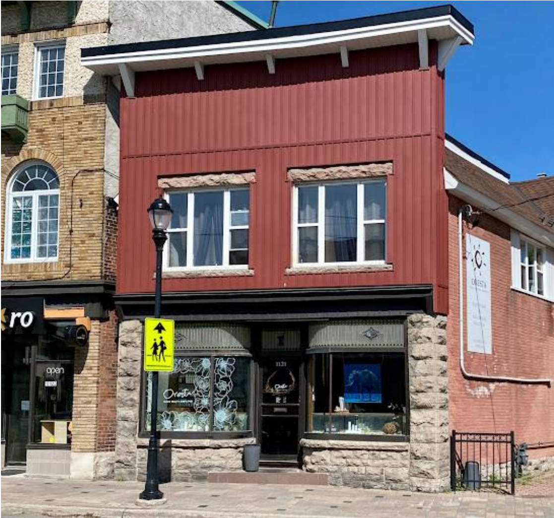
Wellington Street West elevation (Staff Photo, 2024).
