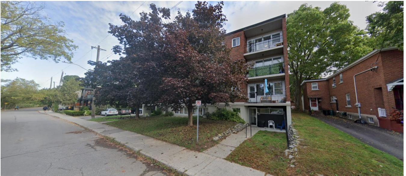
Figure 3: 441 Echo Drive (retrieved from Google Streetview, April 2023)
