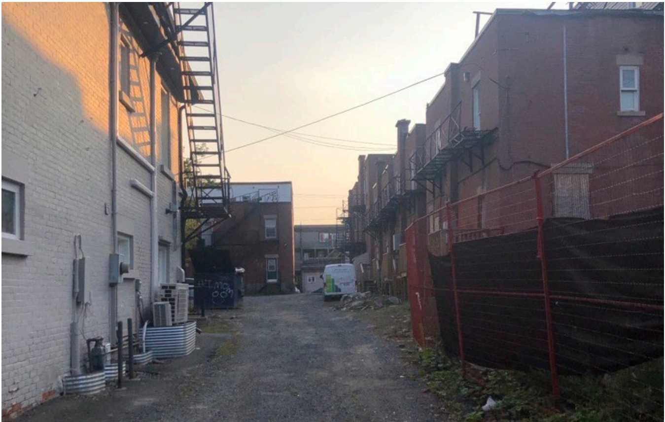
Figure 3: Existing driveway between 146 Osgoode Street and 68 Sweetland Avenue (as viewed from Sweetland Avenue)
