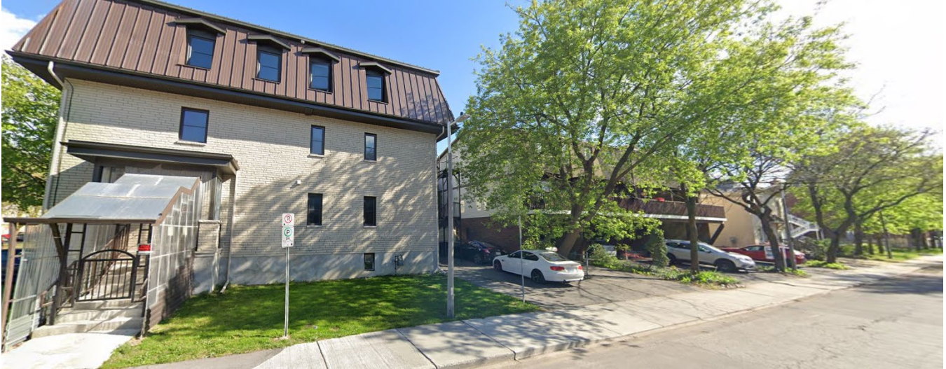
Figure 7: Low-rise residential buildings directly south of the subject property, looking south towards 254 York Street.
