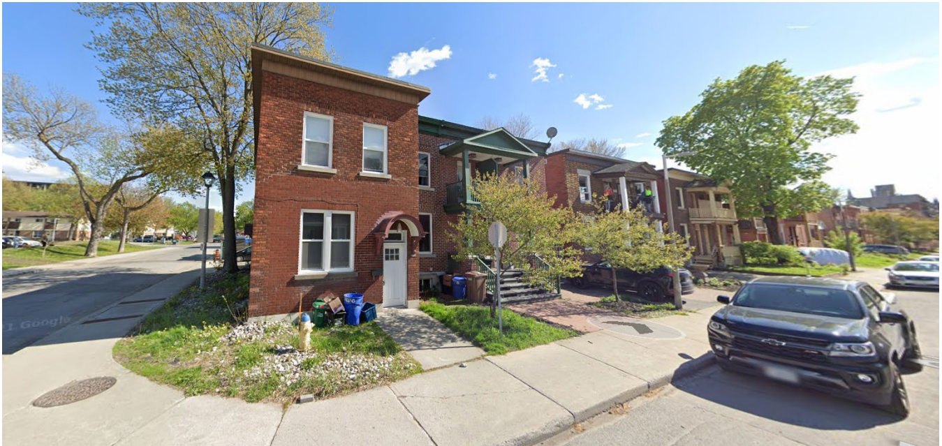
Figure 5: Properties north of the site, looking south towards 300 Clarence Street.
