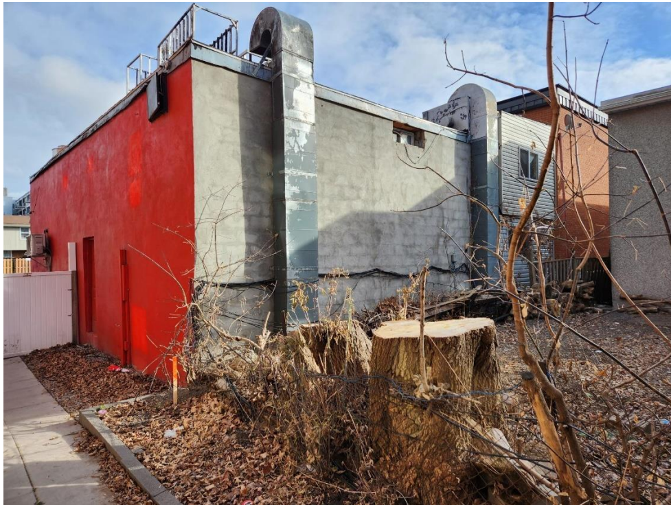
Rear View from Right (North) Side towards Nelson Street
