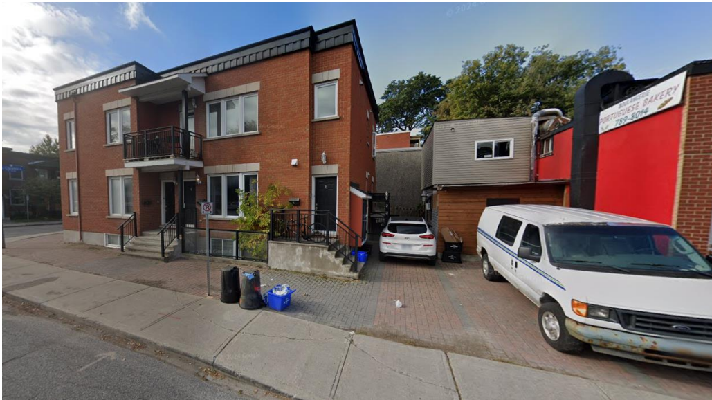
Adjacent Building to Left (South) Side
