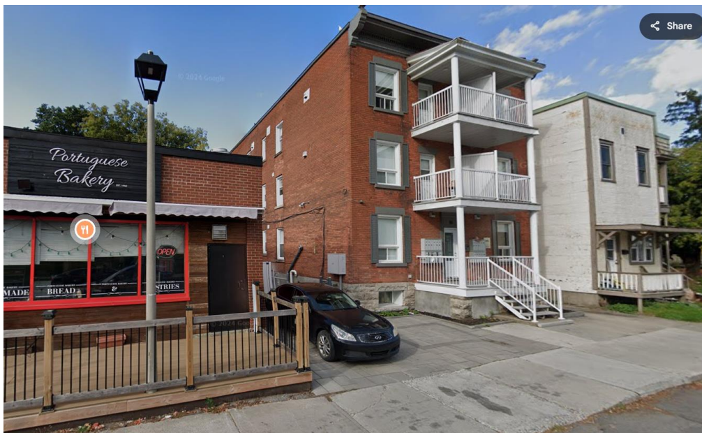
Adjacent Buildings to Right (North) Side
