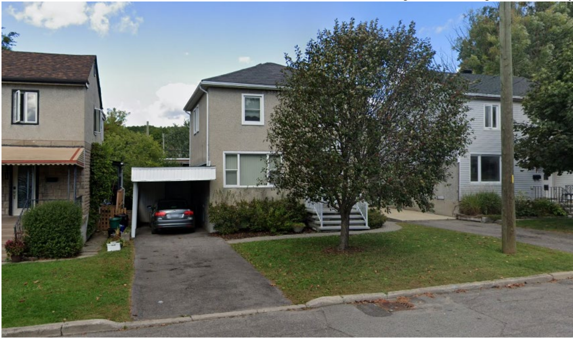
Figure 1: Existing home on Subject Property
