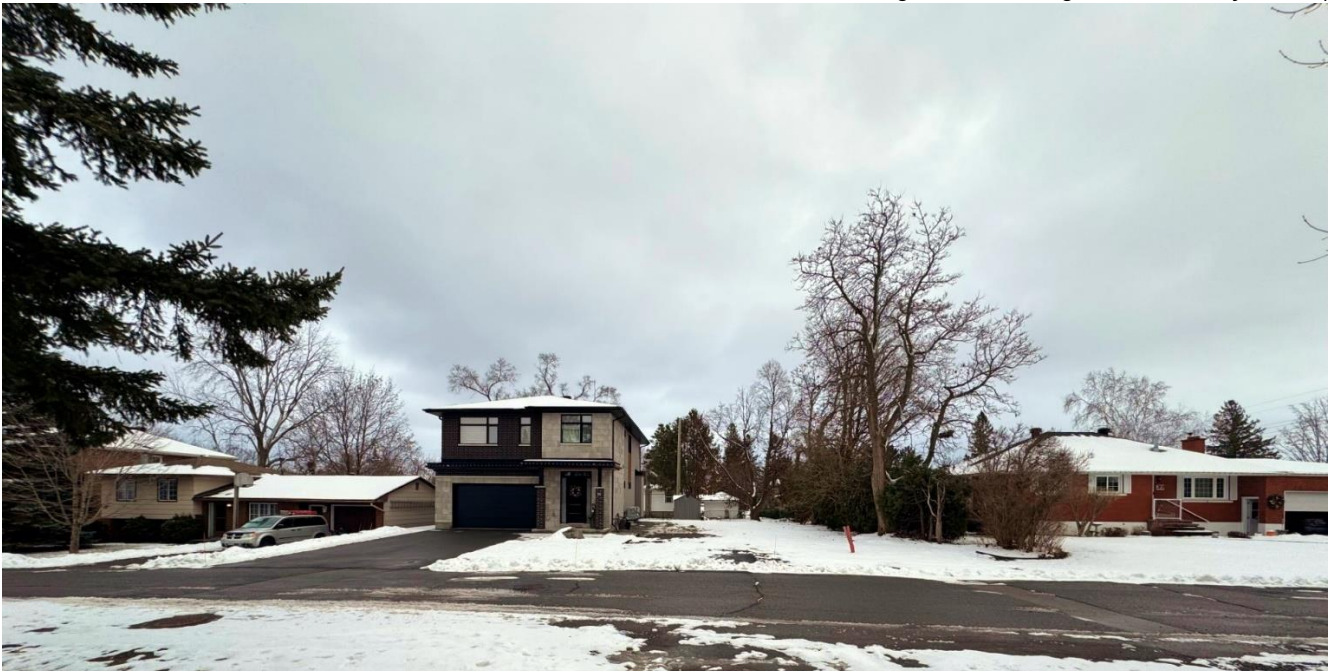
Figure 2: Existing home on Subject Property
