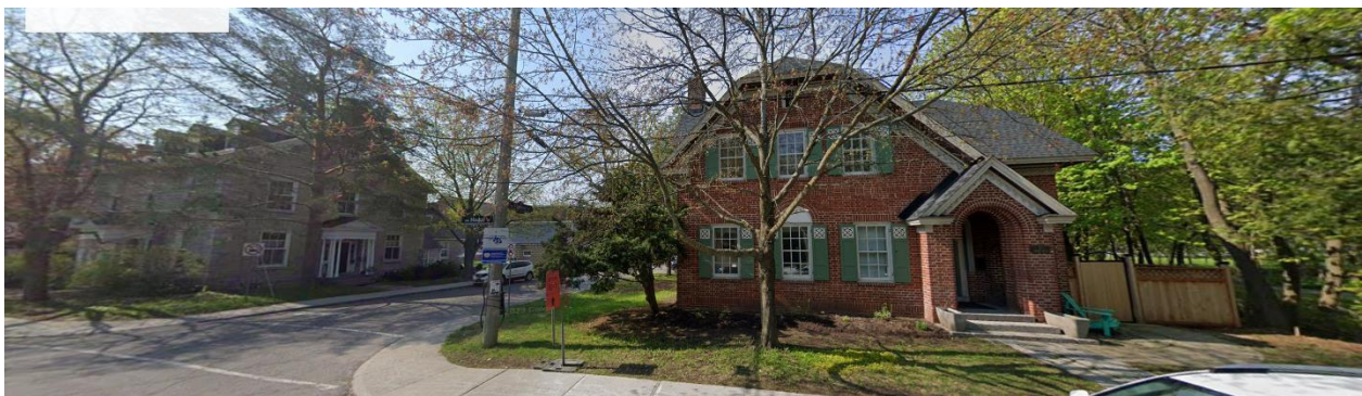
Figure 6: View of 31 MacKay with 71 MacKay across the street on the left. Source Google Maps 2024
