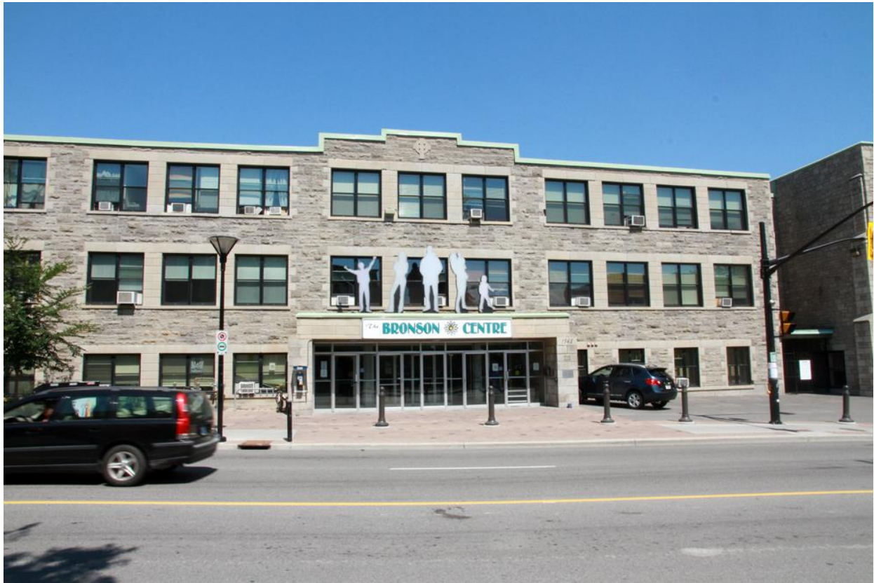
The Bronson Centre, formerly Immaculata High School, on the northeast corner of Bronson Avenue and Lisgar Streets. City of Ottawa , 2016.
