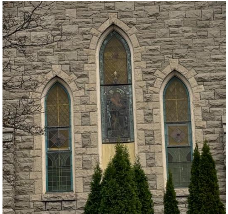
Pointed arched window openings with stained glass windows and rusticated stone voussoirs and sills.
