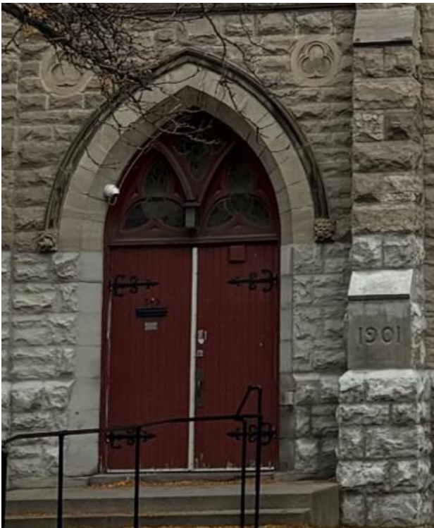
Carved stone hood moulding and label stop.
