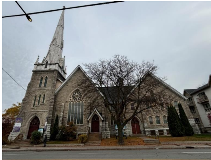
The Bronson Avenue façade of the Erskine Presbyterian Church, showing the original 1901 church (right) and the 1906 addition with the tower and spire (left). City of Ottawa , 2024.
