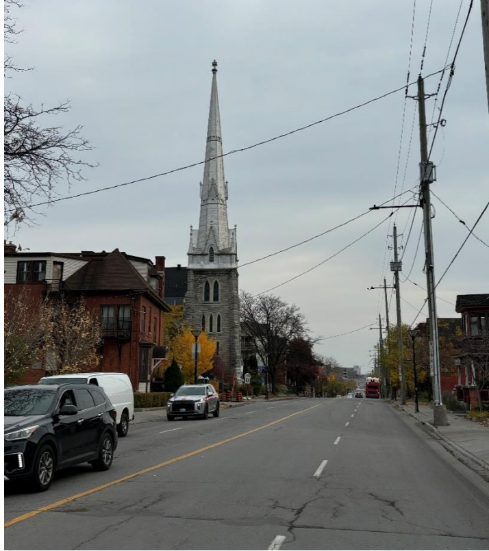
Looking south on Bronson Avenue with various residential building's surrounding the church, Google Maps, 2020.
