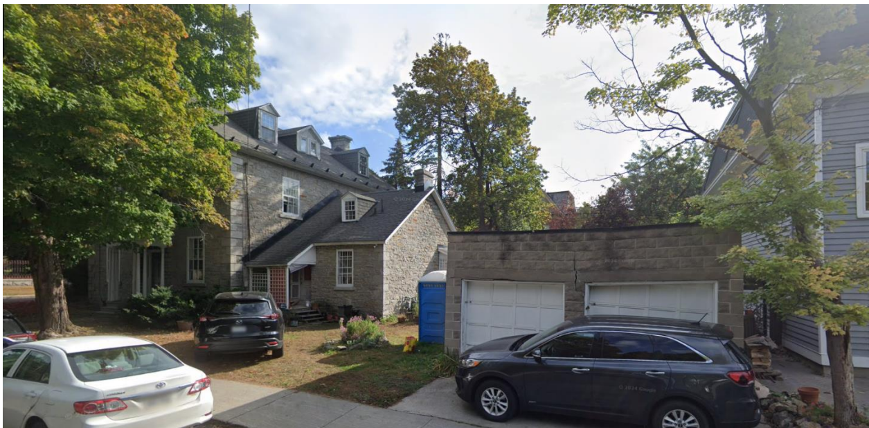
Context photograph of 35 MacKay Street showing the garage to be demolished, Google Streetview
