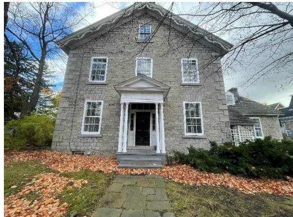
71 Thomas Street Entrance City of Ottawa 2024
