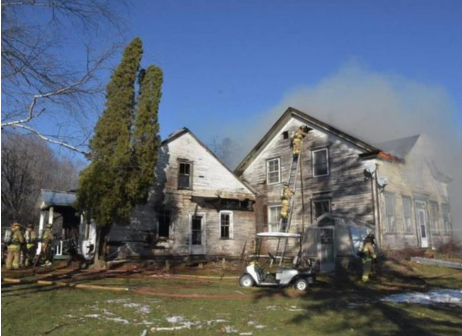
The property during the fire on December 12, 2021. Source: The Ottawa Citizen, December 13, 2021.
