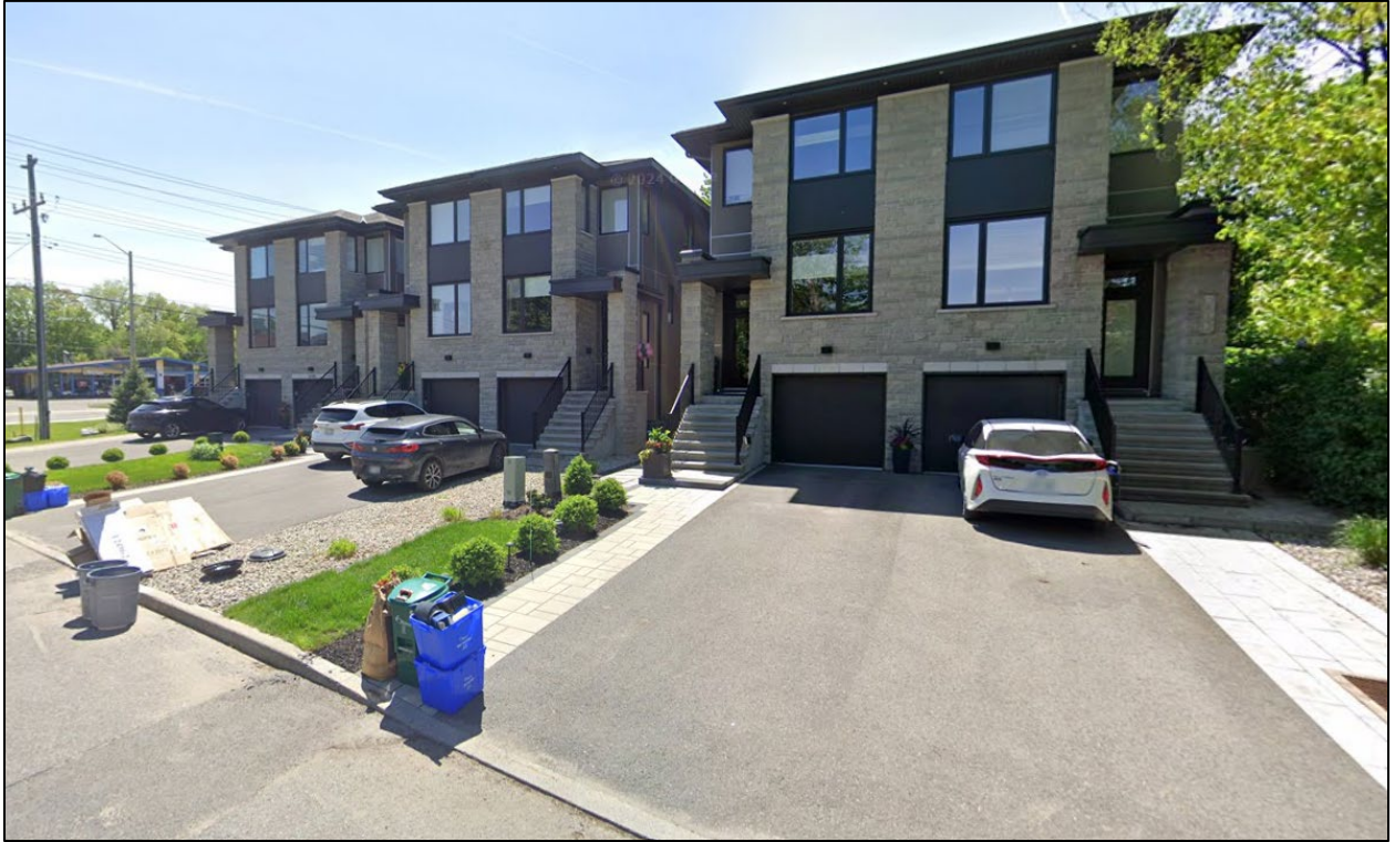
Figure 5 - Infill development occurring on Gravelle Crescent; 2562 – 2572 Gravelle Crescent
