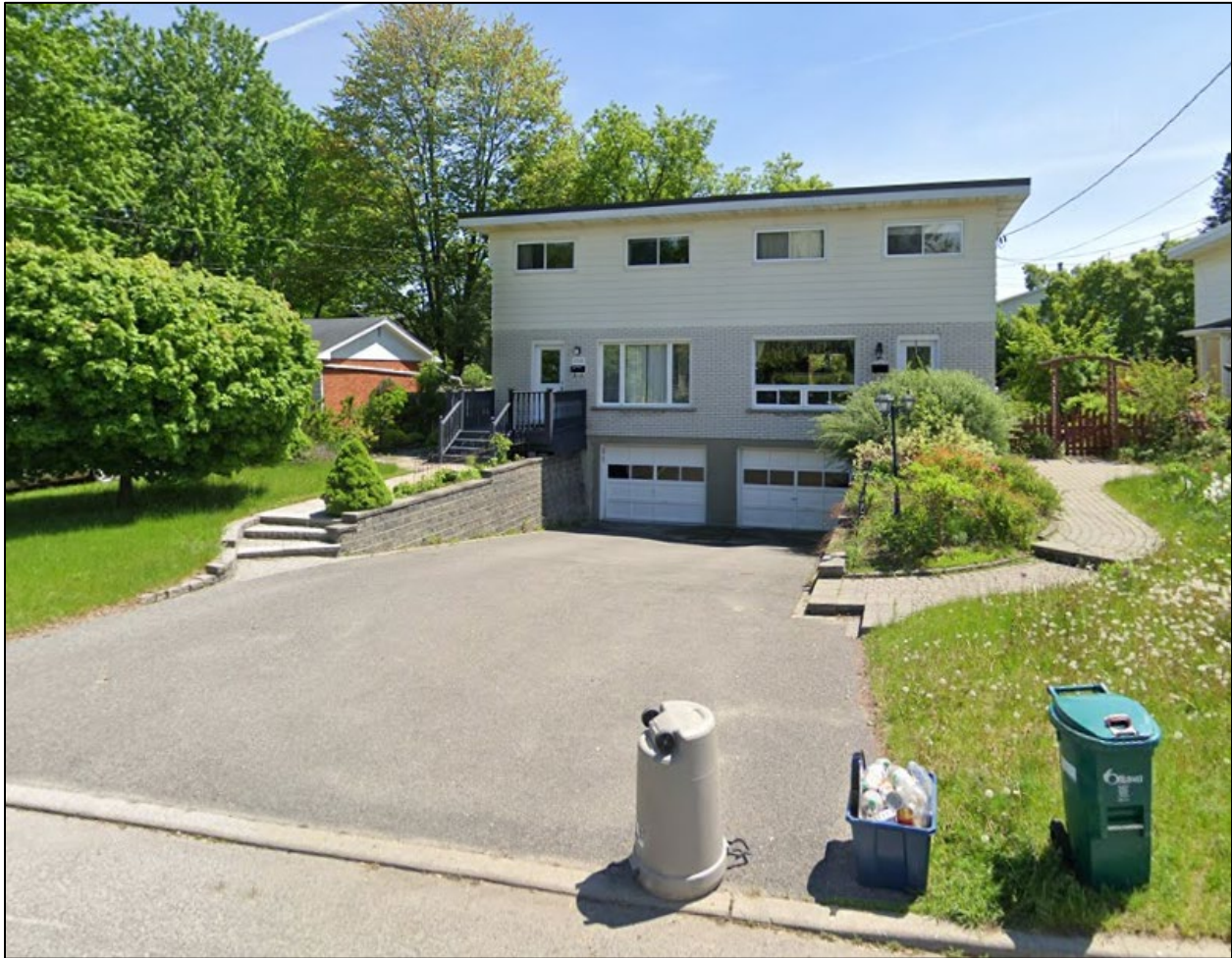
Figure 6 - A variety of housing types exist on the street today; 2518 Gravelle Crescent, semidetached dwelling
