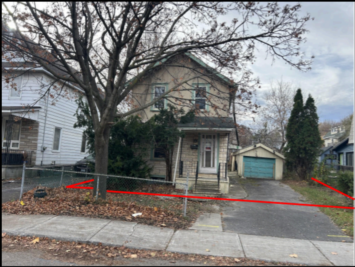
Subject property from Railway indicating the approximate property boundary .
