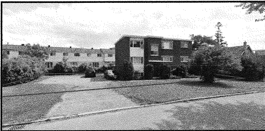
View of 884 Charleswood from Charleswood Ave looking south.
