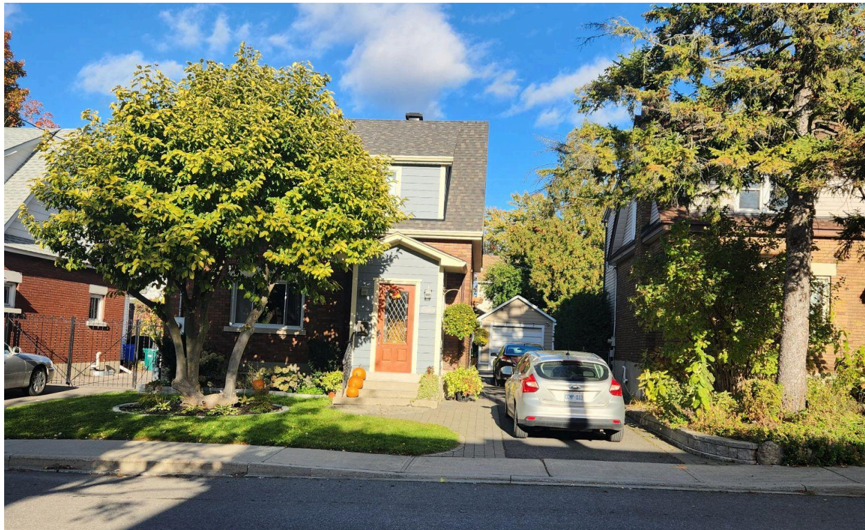
Subject property showing existing dwelling to be demolished, taken Oct 2024.
