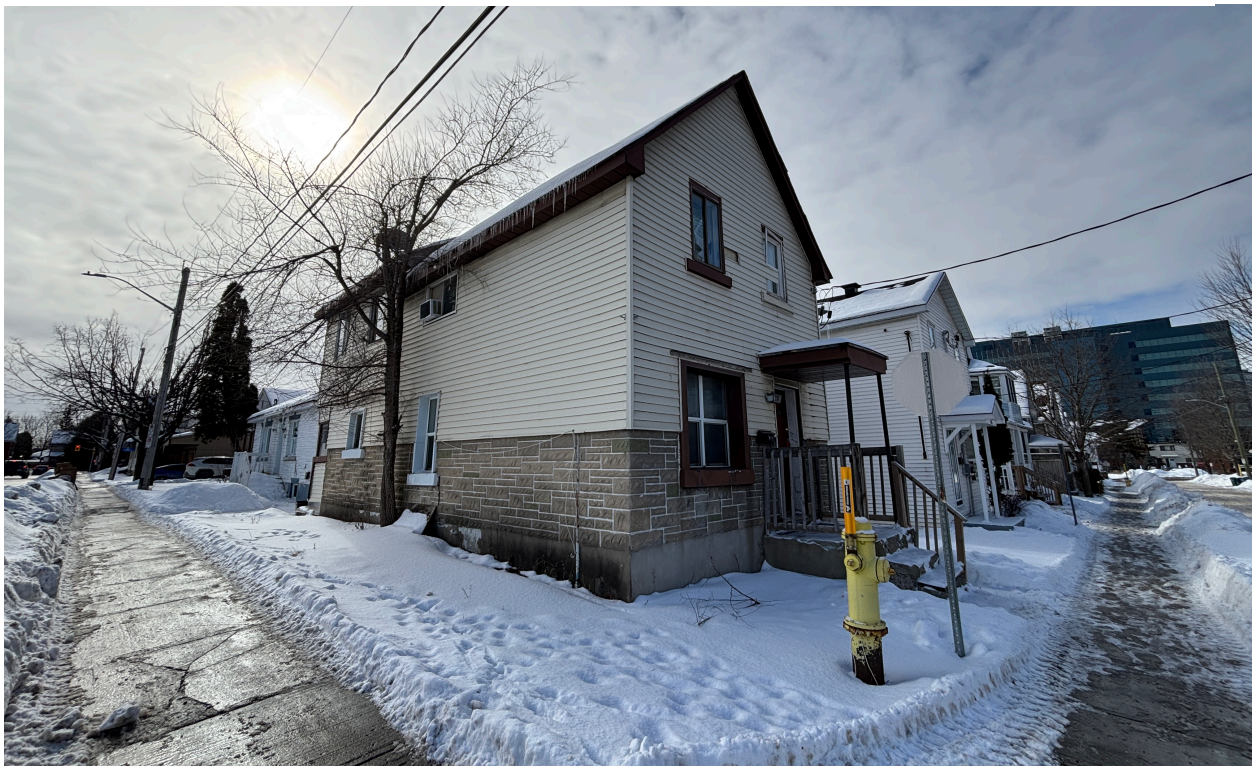
Figure 6: View of the site from the corner of Olmstead and Heritage Maple Way. Both residential buildings will be reconstructed.
