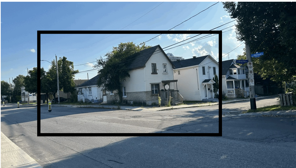
Figure 4: View of the site from the corner of Olmstead and Heritage Maple Way. Both residential buildings will be reconstructed.
