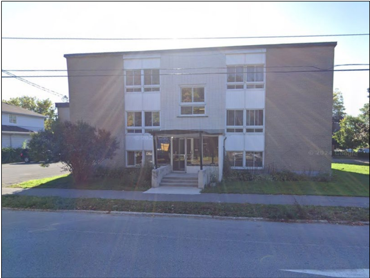
Figure 5 – low-rise apartment at 1240 Shillington Avenue
