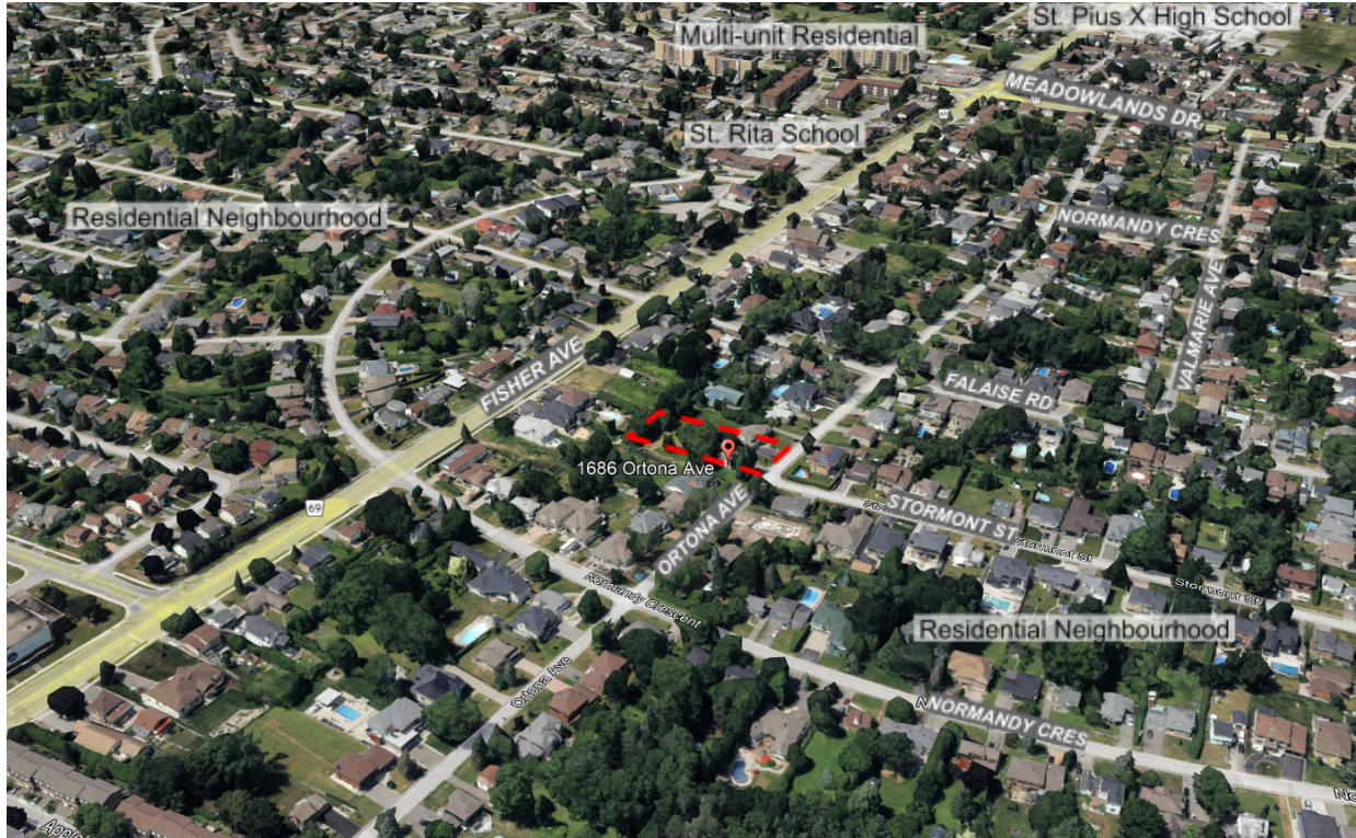
Fig.1. Aerial imagery showing the surrounding context of the subject site, Google Earth.
