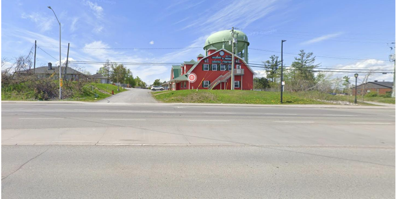
Figure 3: Existing Building on the Subject Site Looking West from Hazeldean Road (Google Maps, May 2023)
