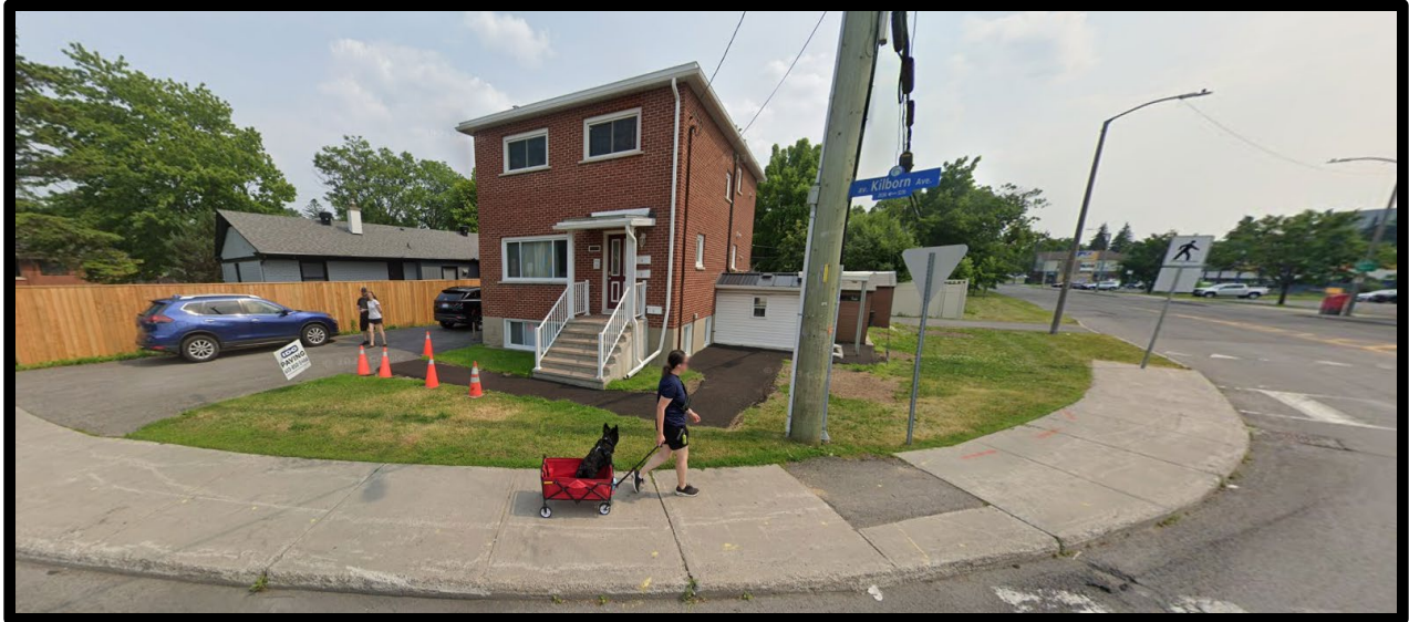
Existing Condition - Frontage of Triplex
