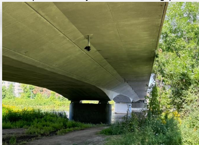
Structure 013010 - Bridge Over Rideau River (CA Transitway Rideau River Bridge)
