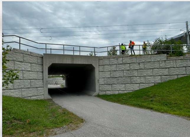
Structure 015720 – Overpass Bayview (MUP U/P Confederation Line E of Bayview Station)
