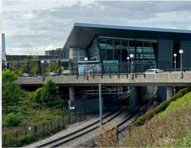
Structure 056660 – Underpass Tremblay (E Twy - Train Stn West Access Rd O/P)
