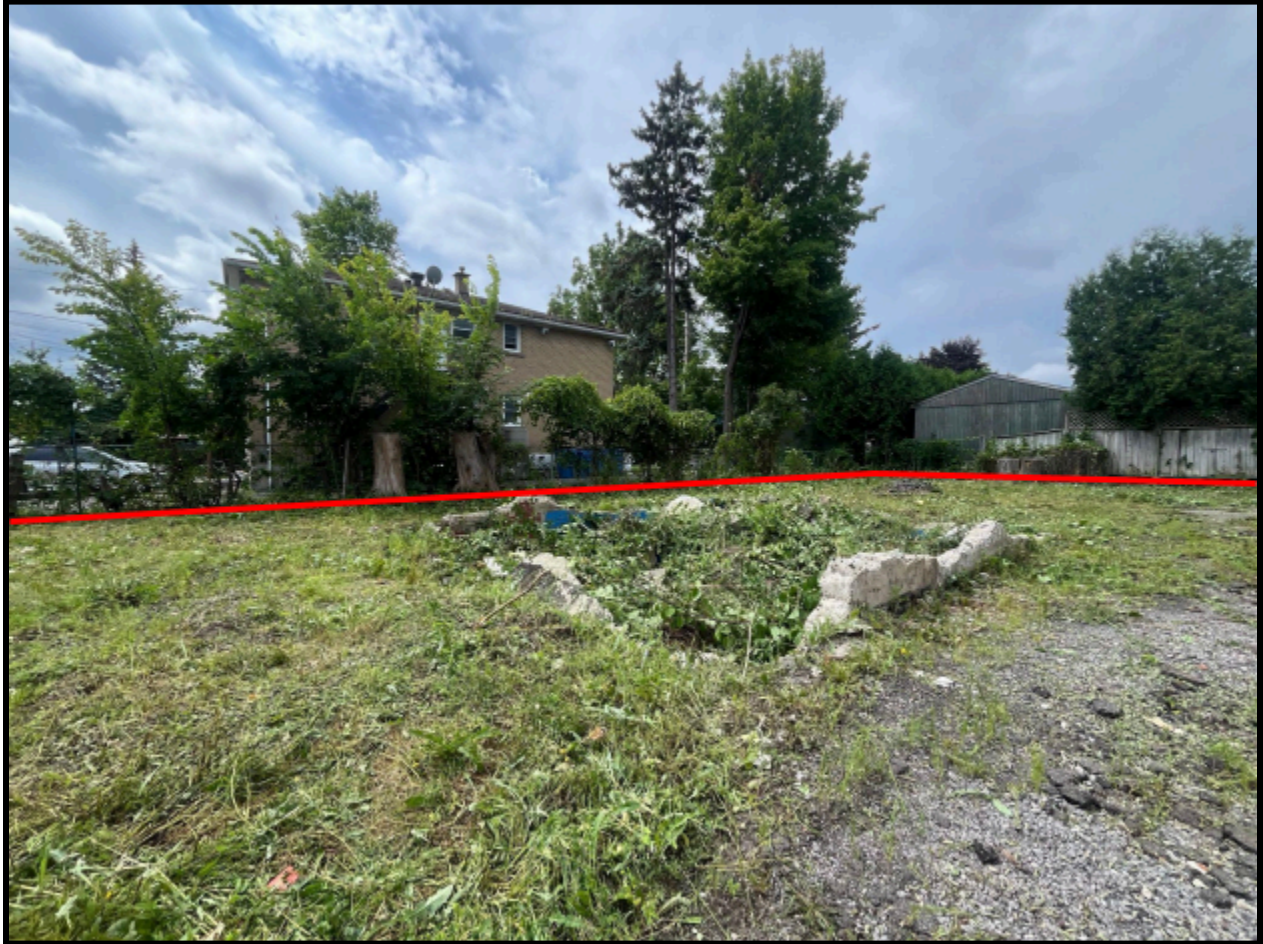
Site photo of the subject property looking southwest at the previous building's foundation. Approximate lot boundary shown in red. (July 2024)
