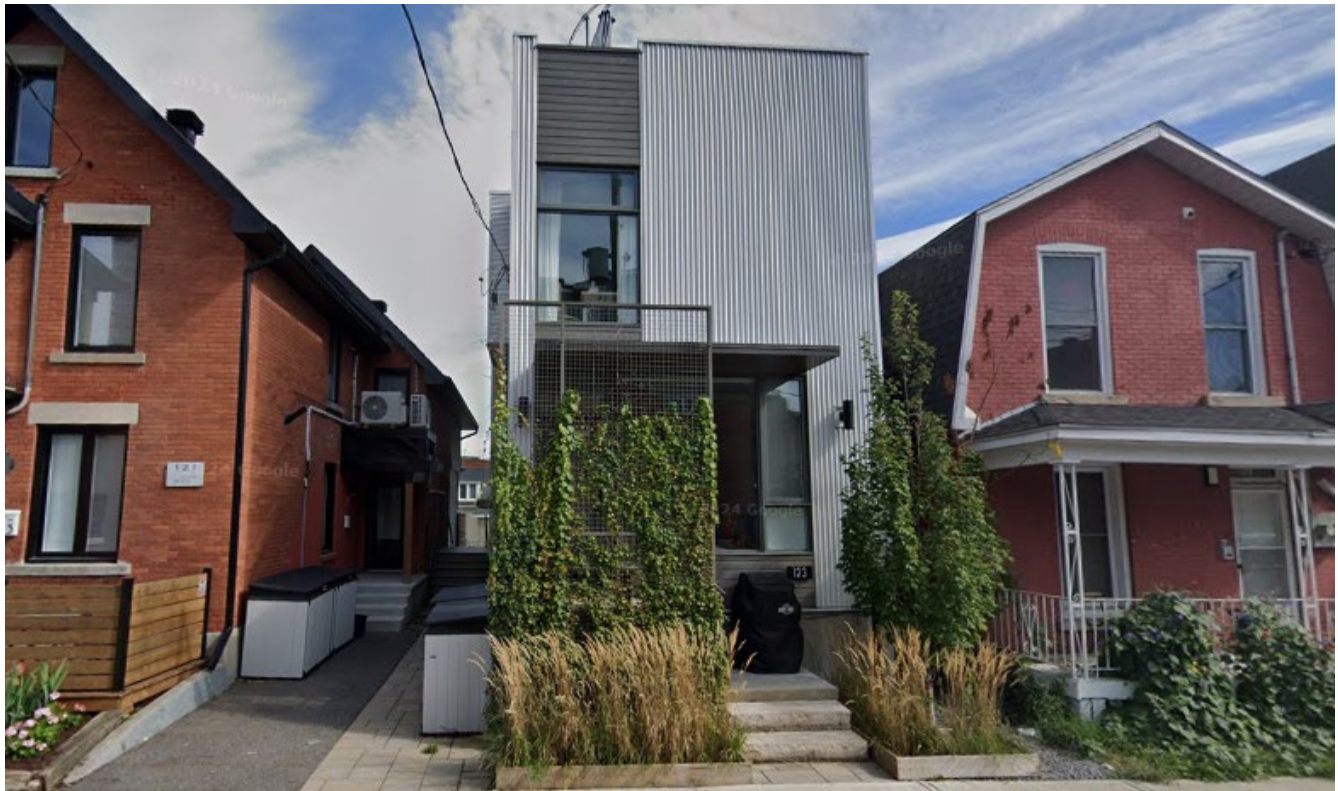
Figure 1. Existing site conditions, front elevation (Google Streetview, 2024)
