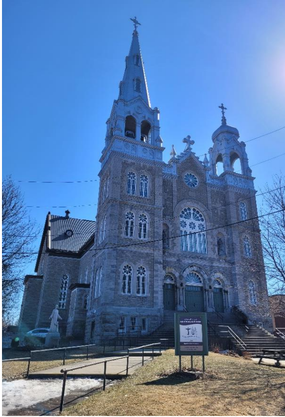
1062 Wellington Street West, northeast façade, Source: City of Ottawa, 2025
