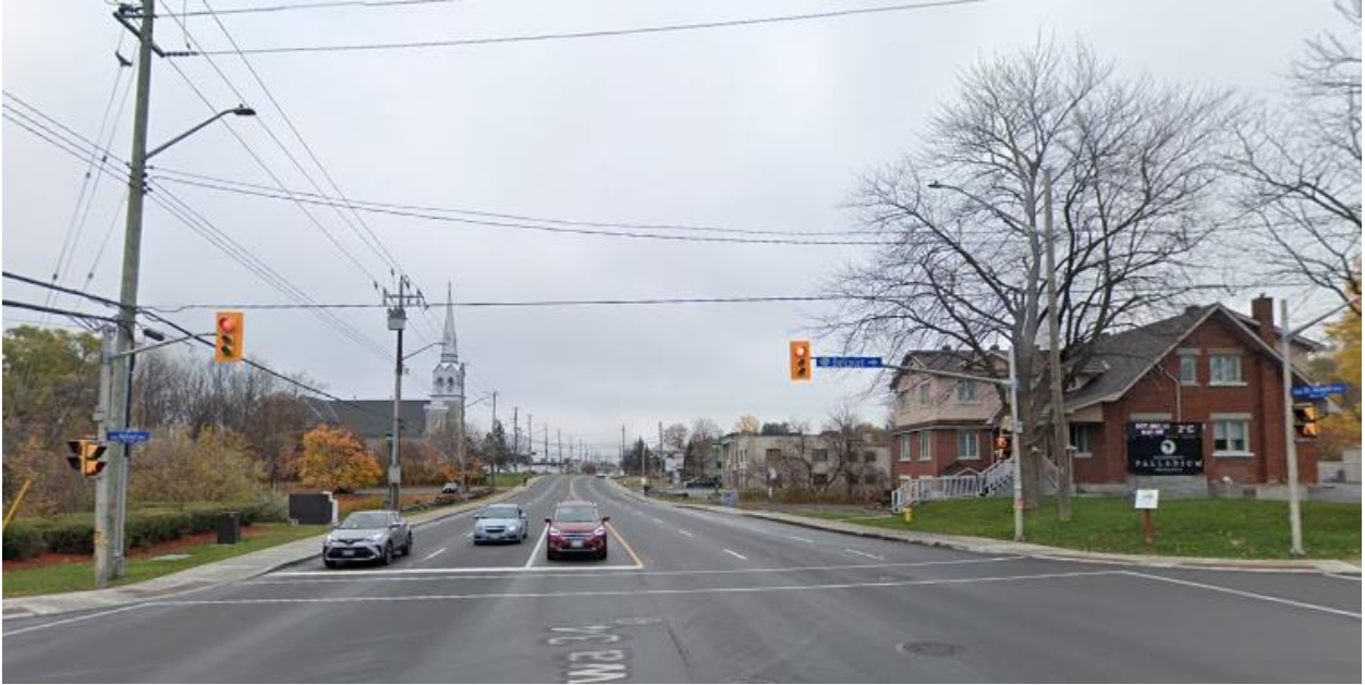
St. Joseph Boulevard looking east at Belcourt Boulevard, Source: Google Streetview, 2020
