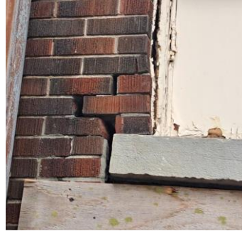
2. Back corner the wall has kicked out and separated requiring extensive temporary bracing.
