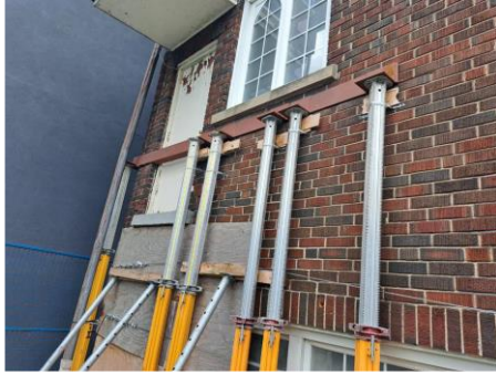
1. Substantial settlement at the corner requiring temporary bracing to prevent collapse of back wall and portion of the east façade.
