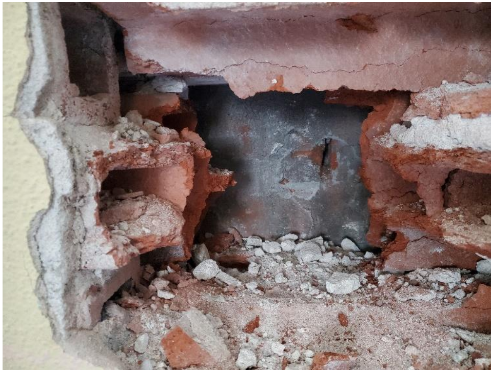
Figure 16: Opening in the Ground Level Wall showing double wythe of hollow terra-cotta with a rough coat and finish coat of plaster on the interior.
