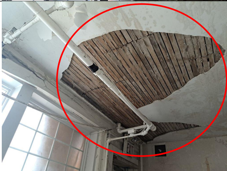
Photo 60 Exposed ceiling due to Gyproc that fell down, and damaged wood frame by water, wood has started to rot
