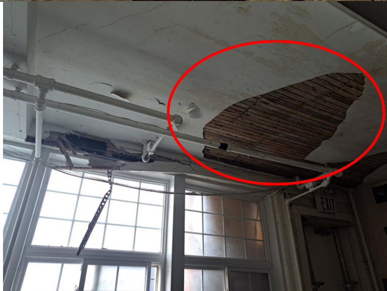
Photo 59 Exposed ceiling due to plaster that fell down, and damaged wood frame by water, wood has started to rot
