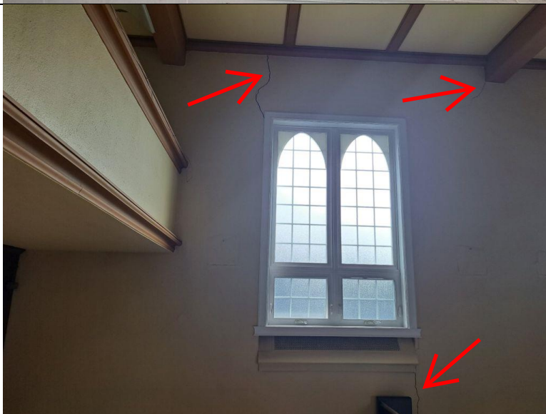
Photo 24 Cracks are noted along the left side (South) wall
