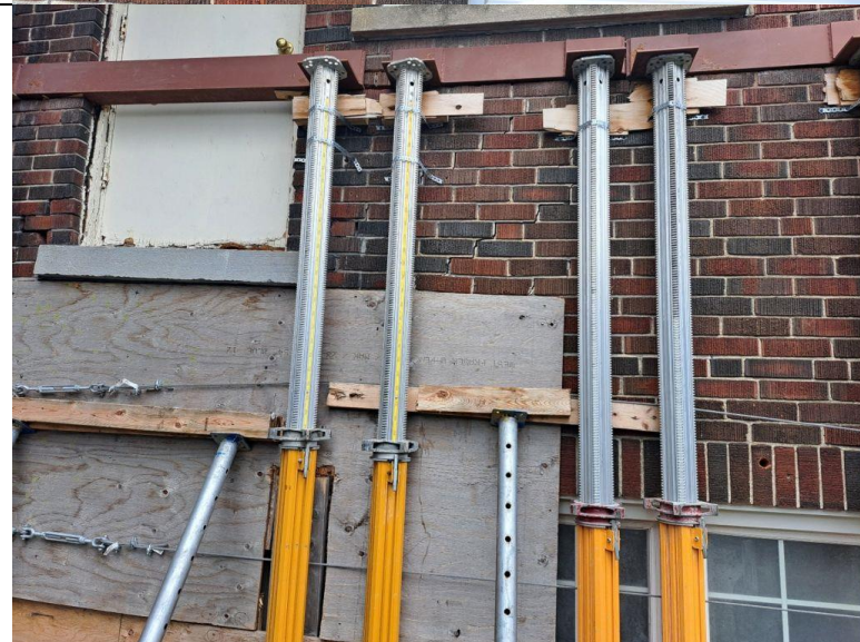
Photo 11 The southeast corner is secured by fastening plywood to the brick and three cables
