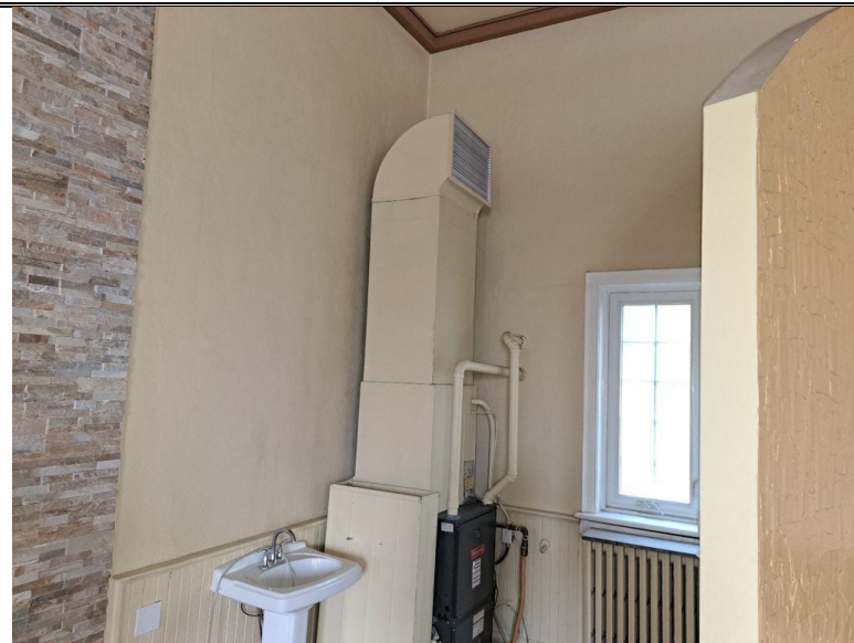
Photo 43 Gas furnace located at the Northeast corner
