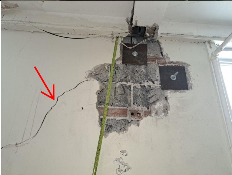
Photo 50 Diagonal cracks of 4mm width
