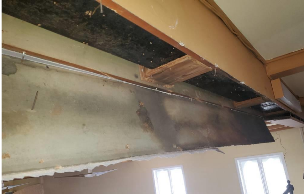
Figure 7: Steel Beam Supporting Roof
