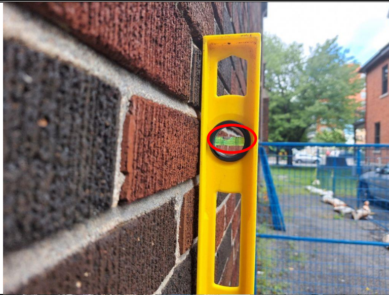
Photo 16 The South wall is leaning to the outside by 1cm for every meter
