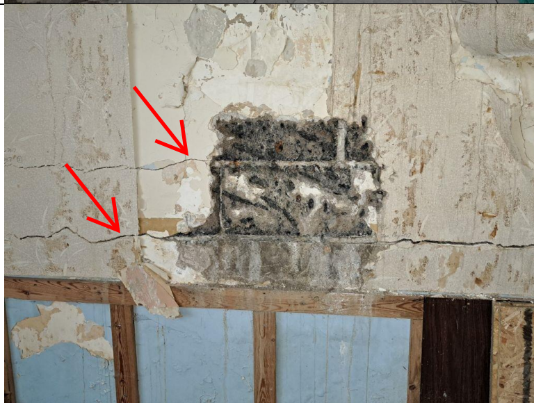
Photo 57 Horizontal crack of at least 5mm width at the rear side wall (East side) at the basement level
