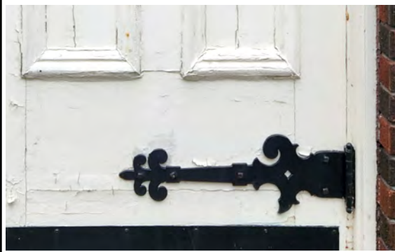
Fig. 13: The bottom of the right door leaf showing a missing section of the metal decorative door hinge, and panel cracks.
