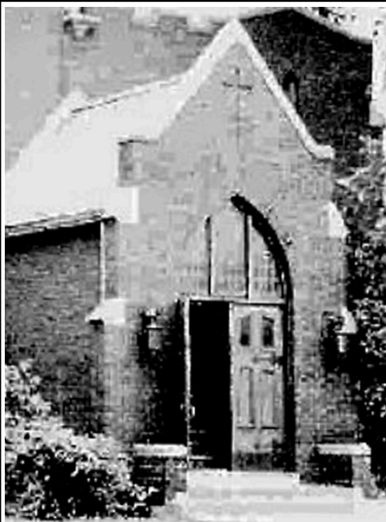
Fig. 14: A detail from a photograph titled, "1929-30 Church Under Construction" showing the main doors and transom. Though it is currently thought that the assembly is non-original, historical evidence shows nearly identical doors, hardware included, implying otherwise. Source: Bibliothèque et Archives nationales du Québec.
