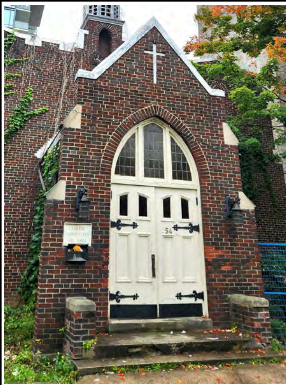
Fig. 15: A September 2024 image of the main doors of the church which strongly resemble those seen in historical images and the building's original blueprints (see Fig. 16). The main difference between this image and the historical image appears to be the transom which is showing wider and more robust mullions and surrounding frame. It is possible that the transom frame has been modified at some point.
