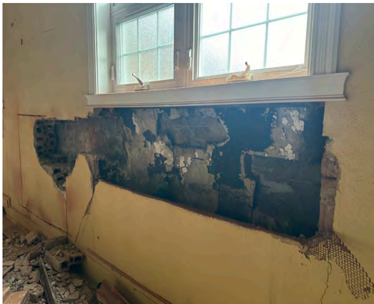
Exploratory opening on the interior, showing wall composition.
