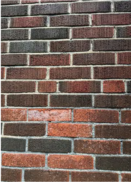
Typical brick condition, with lighter-coloured bricks proving less durable.
