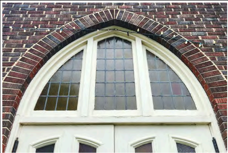
Fig. 19: The exterior face of the Georgian patterned stained and leaded glass transom above the main doors.
