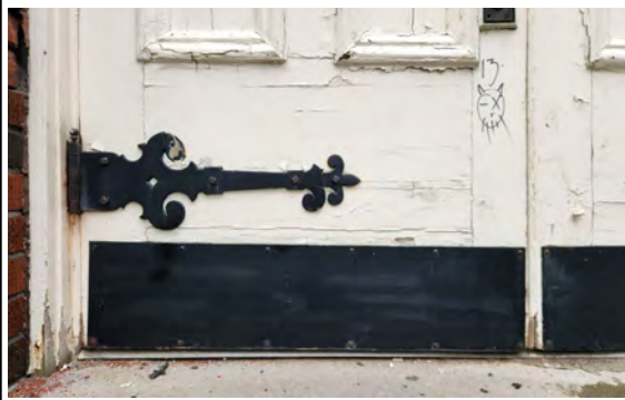
Fig. 12: The bottom of the left door leaf showing existing heavy paint layers failing and corrosion around the metal decorative hinges.
