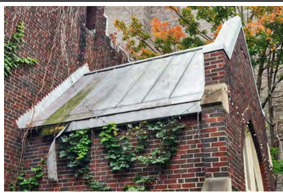
Fig 10: A view of the metal sheeting on the gabled roof over the front, main entrance vestibule. The metal shows soiling and some lifted sections but is overall in good condition.
