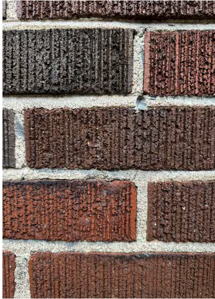
Brick mortar scraped back with steel tool to reveal grey pigmented original mortar.
