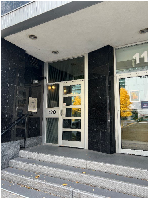
Recessed entrance and original Vitrolite cladding at 120 Holland Avenue, east elevation. City of Ottawa, 2024.
