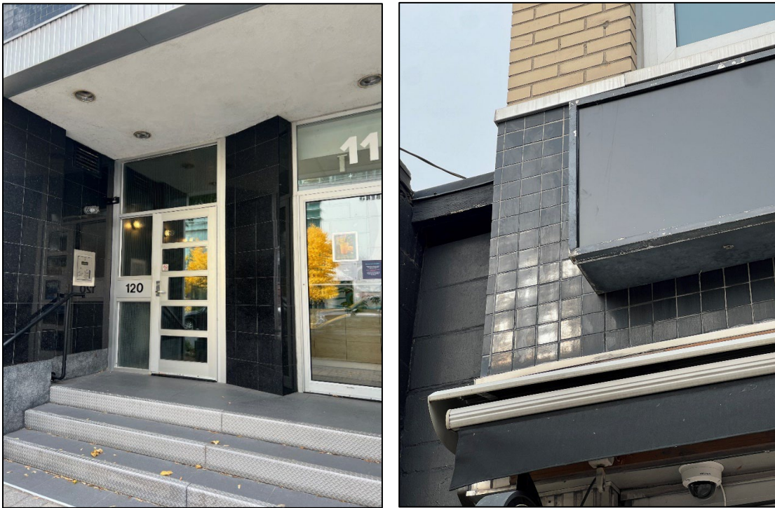
Left: original Vitrolite tile cladding at ground floor main entrance to condominium units (east elevation). Right: black tile cladding above storefront on south elevation, added in 1998. City of Ottawa, October 2024.
