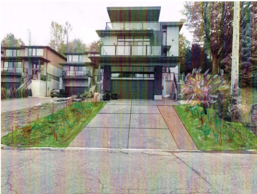
Proposed – Reduced width concrete driveway with saw cuts, separately designed walkway, both with snow melting system.
