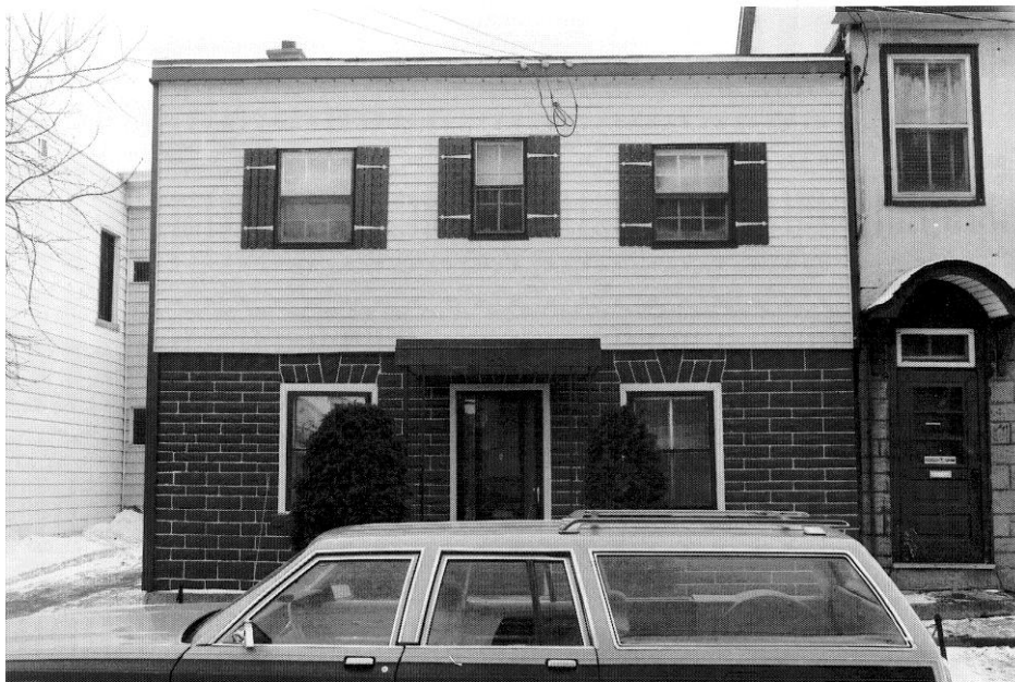
Figure 13: A view of 168 Murray Street as altered circa 1965. The house has been remodelled with a flat roof, second floor added, and three windows replacing the dormers. The exterior was reclad in an angel stone on the ground floor and aluminum siding on the upper floor. A canopy over the front door has been added. Source: City of Ottawa Heritage Survey Forms 1991.
