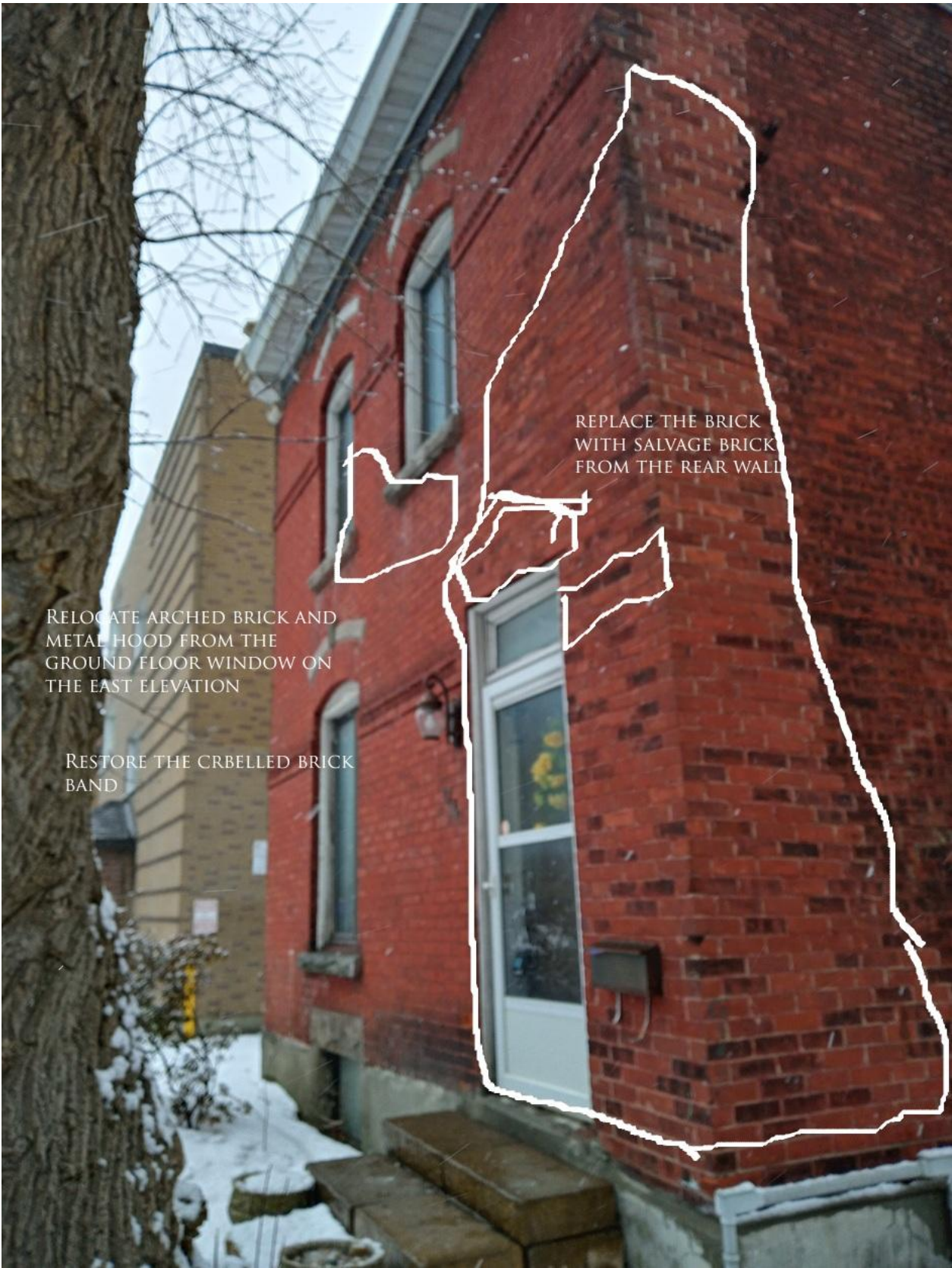
Figure 45: As -found image with areas requiring repair and restoration highlighted in white.
