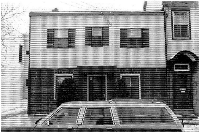
Figure 4: A 1991 view of the house documents the substantive alteration from its original one-and-one half storey side gable roof with gabled dormers facing the street. The house has been remodelled with a flat roof, a second floor added, and three windows replacing the dormers. The exterior was reclad in an angel stone on the ground floor and aluminum siding on the upper floor. A canopy over the front door has been added. Source: City of Ottawa Heritage Survey Forms 1991.
