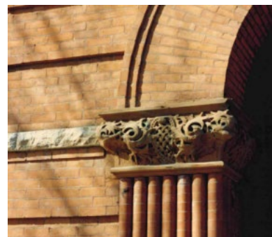
Carved sandstone and curved brick pilasters of the main entrance arch. 1991, City of Ottawa.
