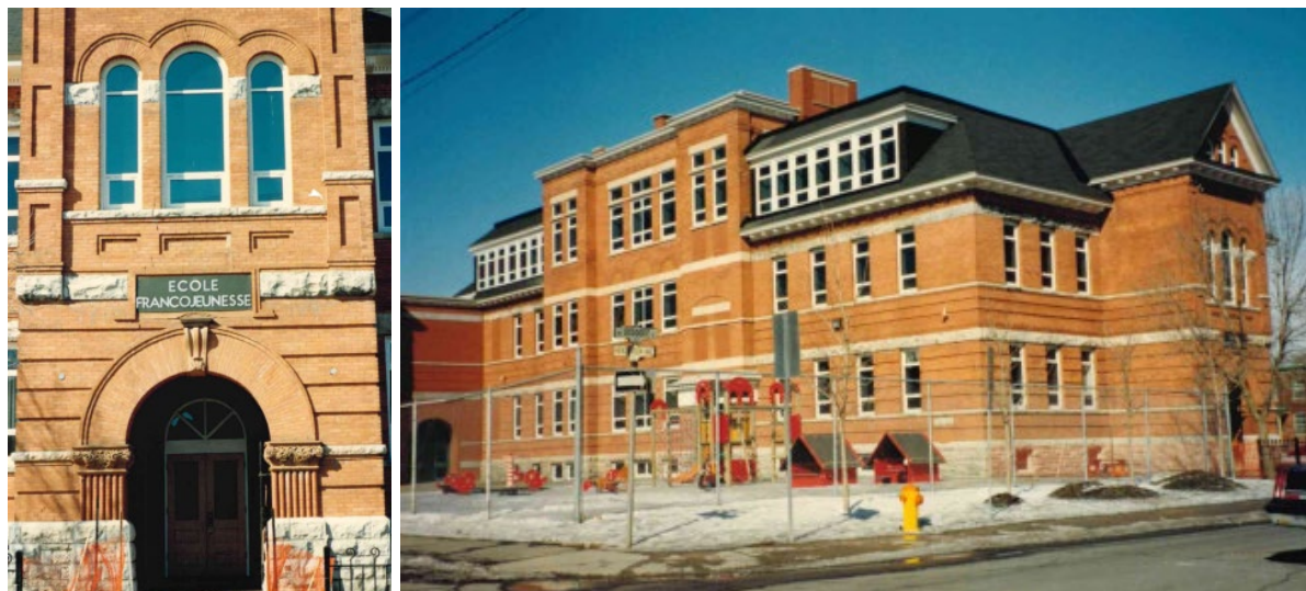
Left: Detail of the frontispiece displaying the school name. Right: A chimney marks the rear wall of the original school. Images 1991, City of Ottawa.
