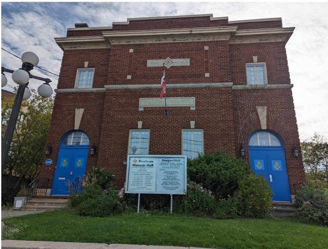
Front façade of 430 Churchill North, looking west. (Source: City of Ottawa, 2023)
