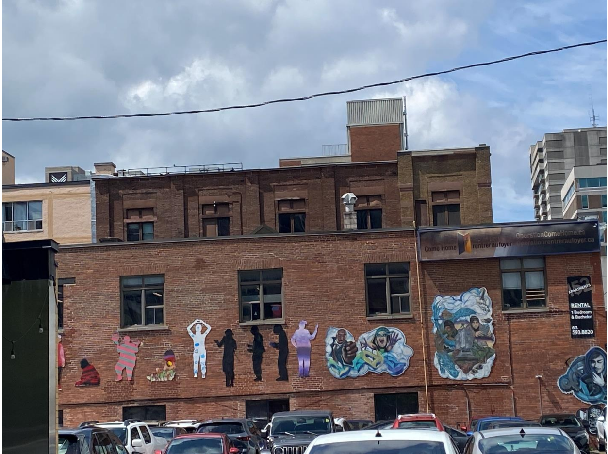
East façade (partially obstructed by 150 Gloucester Street)
