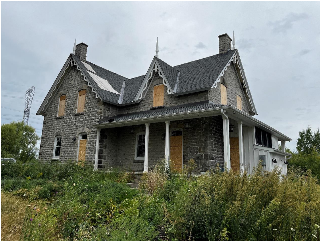
Current condition, City of Ottawa, 2025
