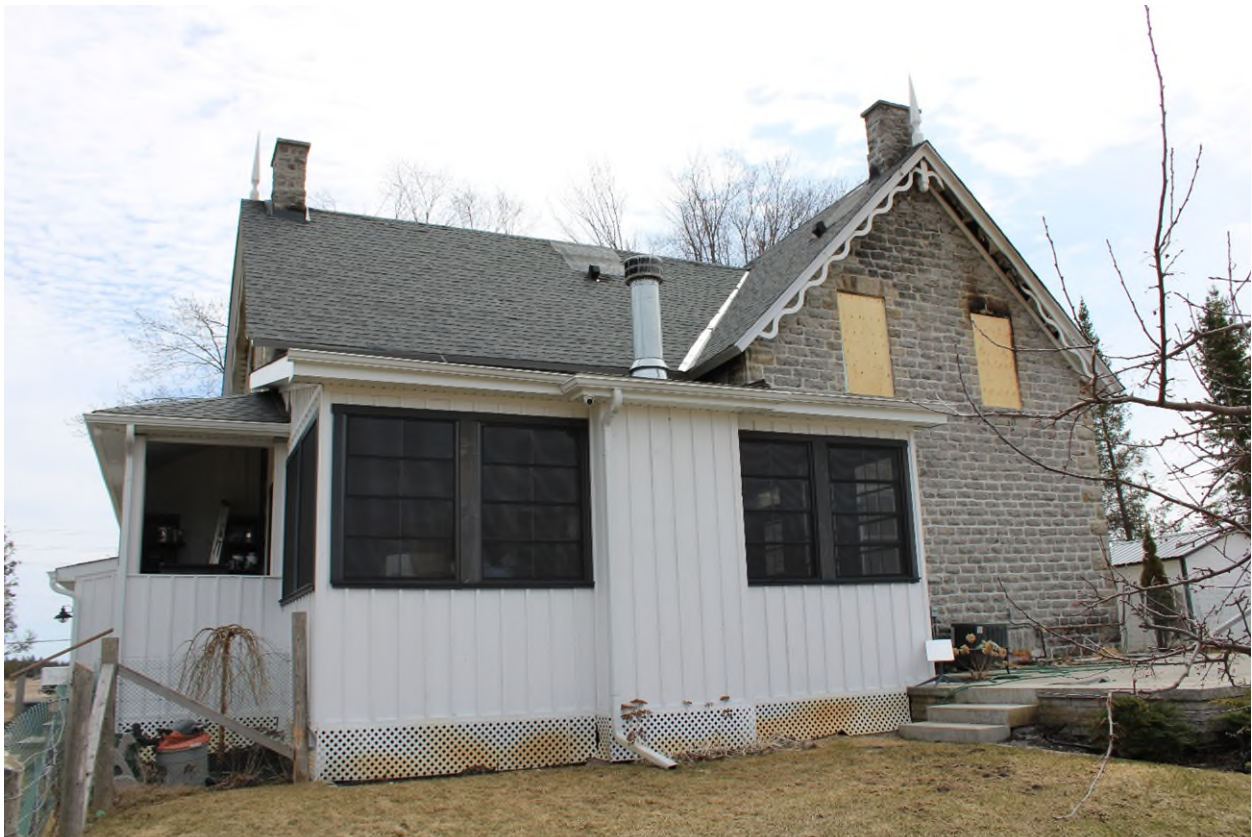
Photograph 03 –North (Rear) Elevation – Taken by Pario on April 14, 2025.
