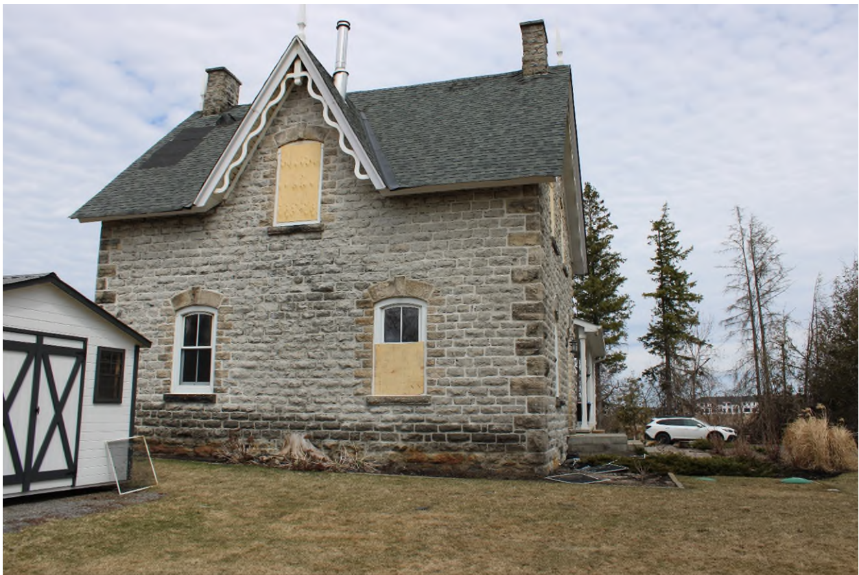
Photograph 02 – West (Side) Elevation – Taken by Pario on April 14, 2025.
