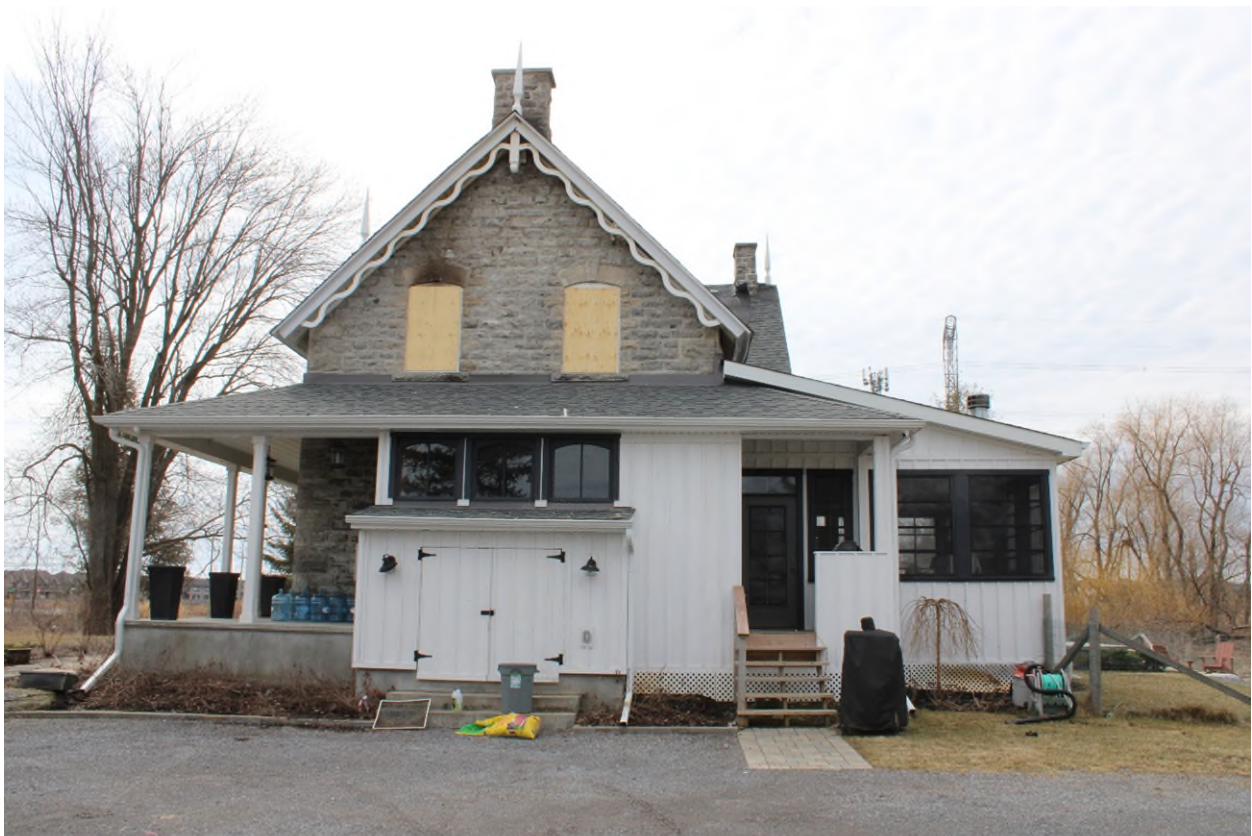
Photograph 04 –East (Side) Elevation – Taken by Pario on April 14, 2025.
