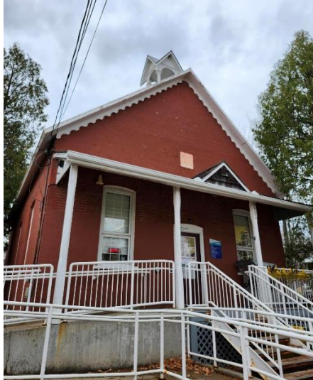
Front façade of 8682 Bank Street showing entrance, veranda with pediment, bargeboard under front gable and stone foundation. Source: City of Ottawa Staff (2024).
