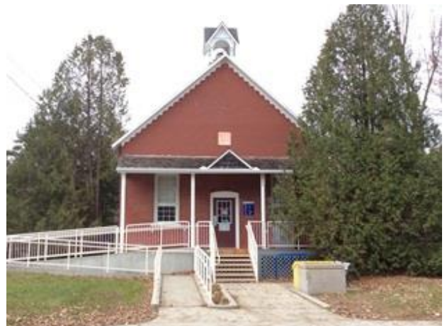
Front façade after addition of accessibility ramp. Source: City of Ottawa (2019).
