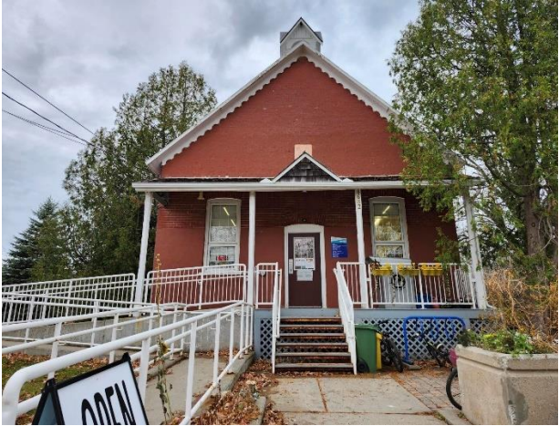
East (front) façade. (City of Ottawa Staff, 2024)
