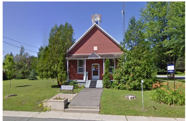
Front façade prior to addition of accessibility ramp. Source: Google Streetview (2009).
