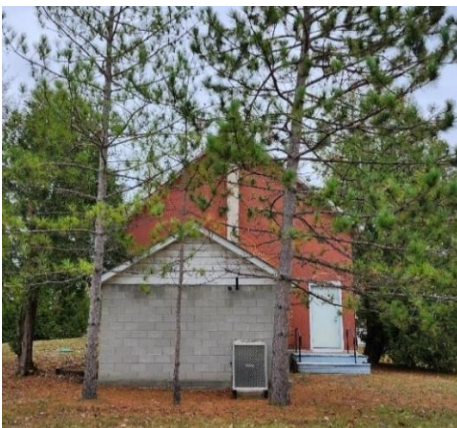
Back of building facing west. Source: City of Ottawa Staff (2024).
