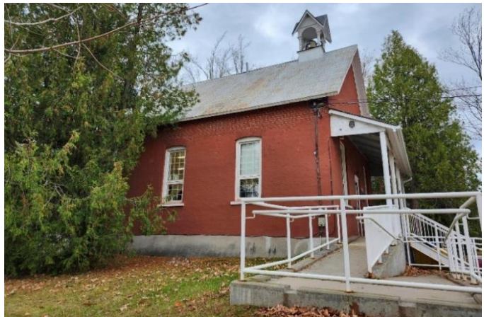
Side of building facing south. Source: City of Ottawa Staff (2024).
