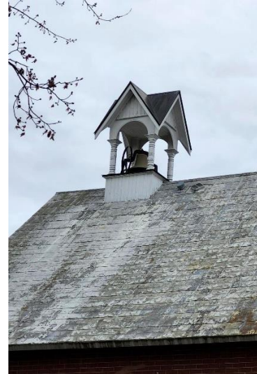
Wooden belfry and metal roof. Source: City of Ottawa Staff (2024).
