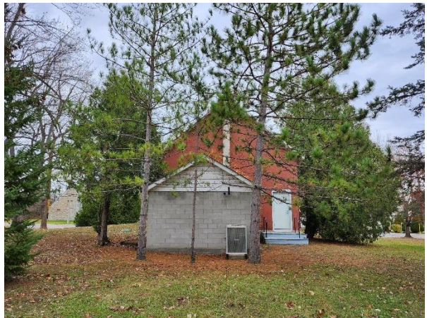
West (rear) elevation. (City of Ottawa Staff, 2024)
