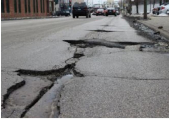
Image 16: Several potholes are seen on an asphalt road (left) and a newly installed rain garden (right).
