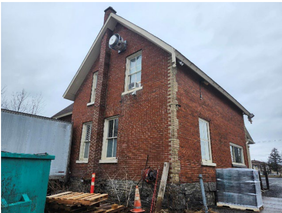
Rear (west) elevation of property
