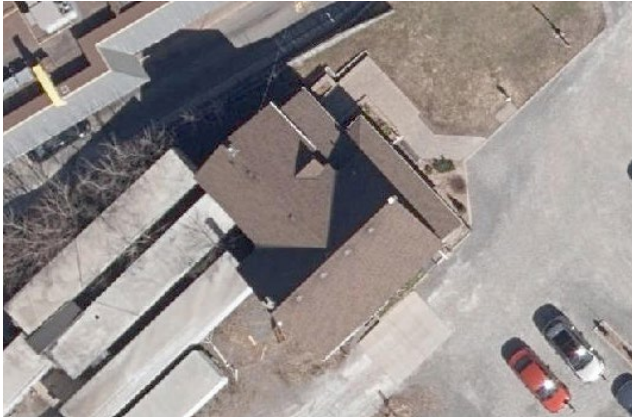
Aerial view of the property at 2400 Bank Street. Source: Google Maps (2021)
