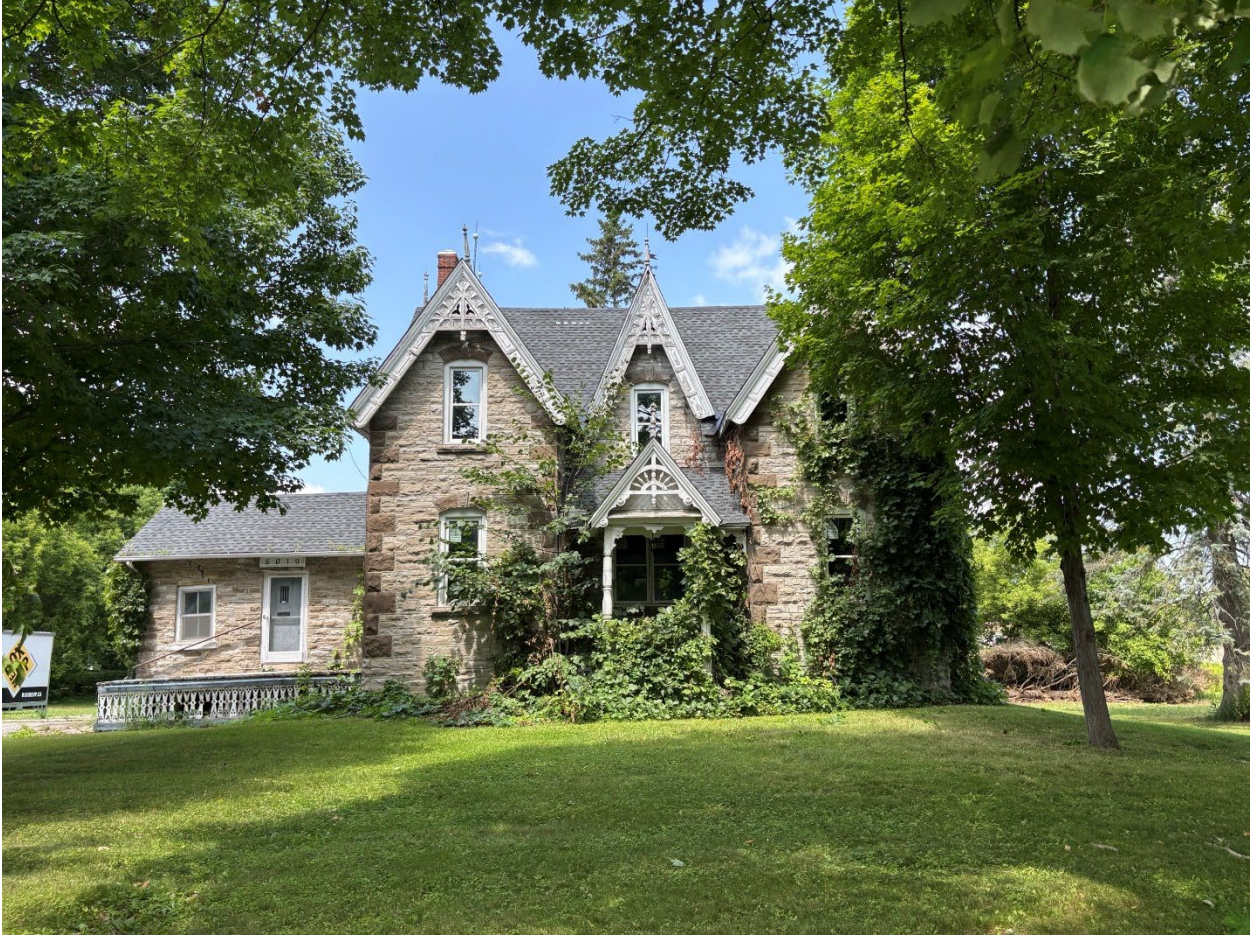
Photo B: South (front) façade (Source: City of Ottawa, 2025.)
