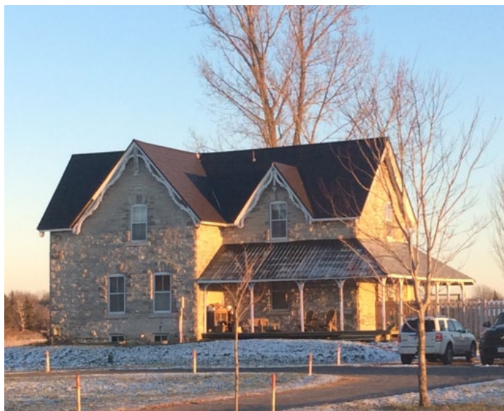
5100 Fallowfield Road, constructed 1886. City of Ottawa , 2018.
