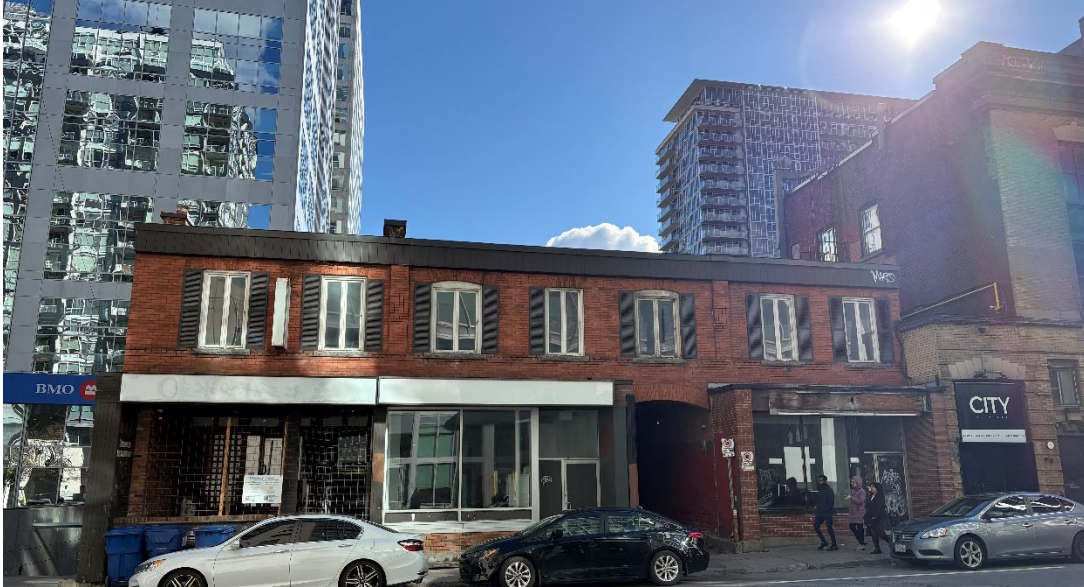
Image 3: 208 Slater Street, City of Ottawa 2025
