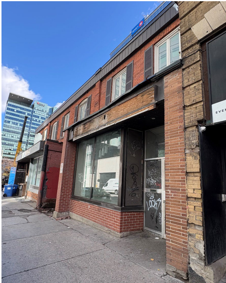
Image 4: 208 Slater Street, City of Ottawa 2025
