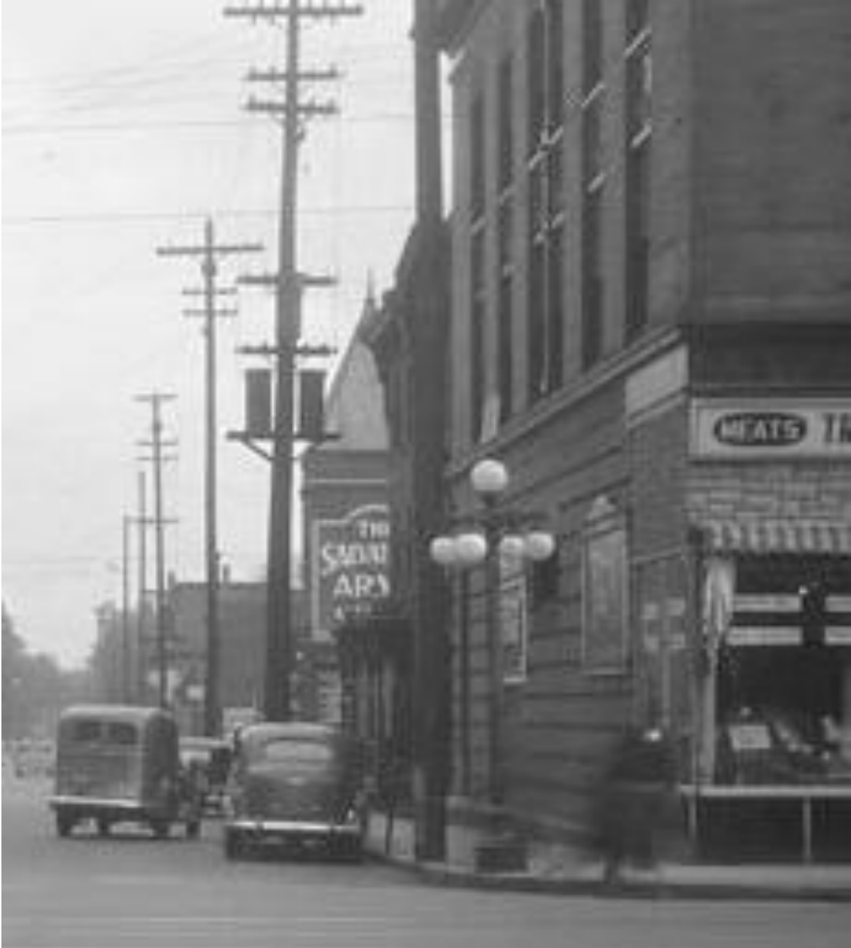
Figure 14: The blow-up of the 1938 photo provides a slightly better view of 208-212 with what appears to be two entrance porches to Units 208 and 210 enclosed with a roof structure that extends to the property line. The porches have decorative spindled columns and fret-work. The building is three storeys in height and the galvanized metal cornice reflects the articulation of the two projecting pilasters that divide the 3-bay façade with a 2:3:2 fenestration pattern. Source: Archives Canada Public Works 1938 photograph. To view on a high-resolution monitor visit http://data2.archives.ca/e/e438/e010934846-v8.jpg
