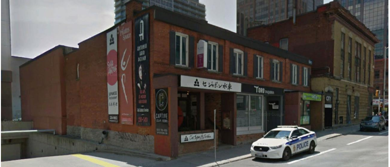
Figure 7: View looking west on Slater to the development site. Note the projecting brick walls enclosing the storefronts. Note the east wall (left) and the stone foundation walls that delimit the original built plan. The rear addition evident to the left of the photograph was completed post 1965. Source: Google Earth
