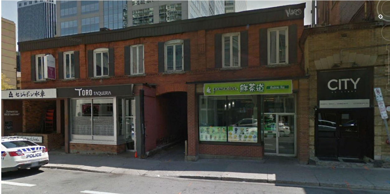
Figure 15: View of the 3-bay façade articulated with projecting pilasters that group the bays into a 2:3:2 fenestration pattern. The central bay is further articulated with a central flat headed window flanked by two wider windows with segmental brick arches. Source: Google Earth.
