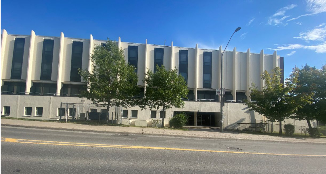
North Façade (Source: City of Ottawa, 2025)
