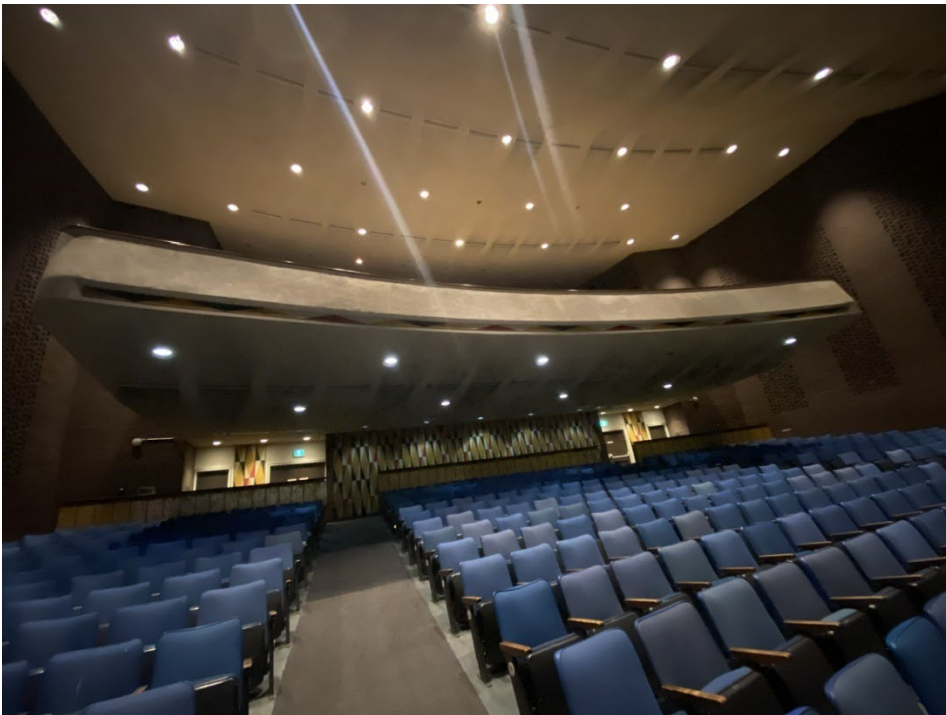
Auditorium Interior – Balcony Detail (Source: City of Ottawa, 2025)
