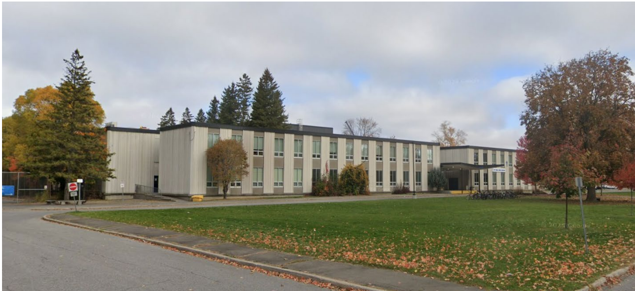
Sir John A. MacDonald High School, now the St. Paul Catholic High School at 2675 Draper Avenue. (Source: Google Maps, 2024).
