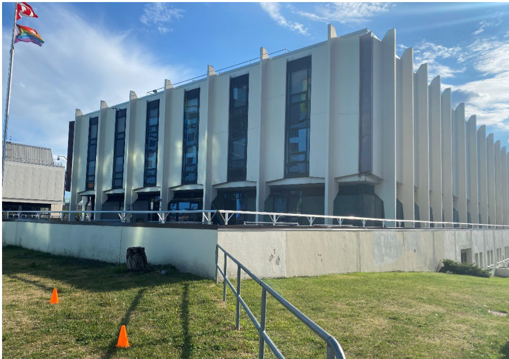
Classroom Detail (East and North Façades) (Source: City of Ottawa, 2025)
