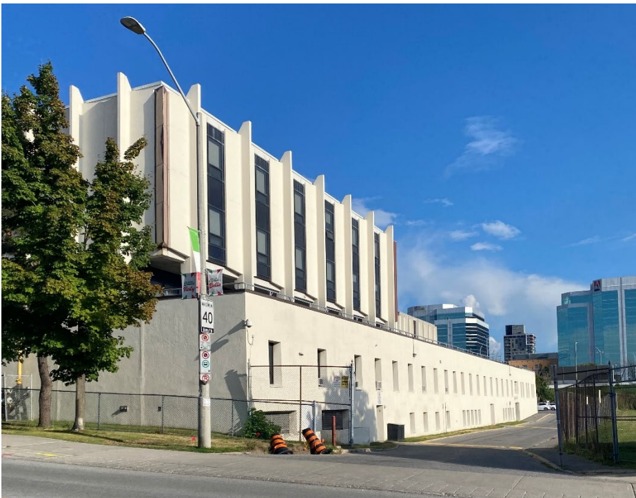
West Façade (Source: City of Ottawa, 2025)
