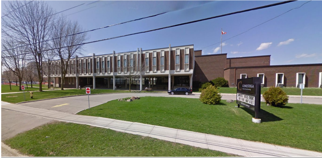
Conestoga College, Waterloo Campus (Source: Google Maps, 2009)
