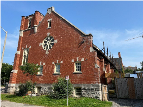
Figure 4: North Façade (Source: City of Ottawa)
