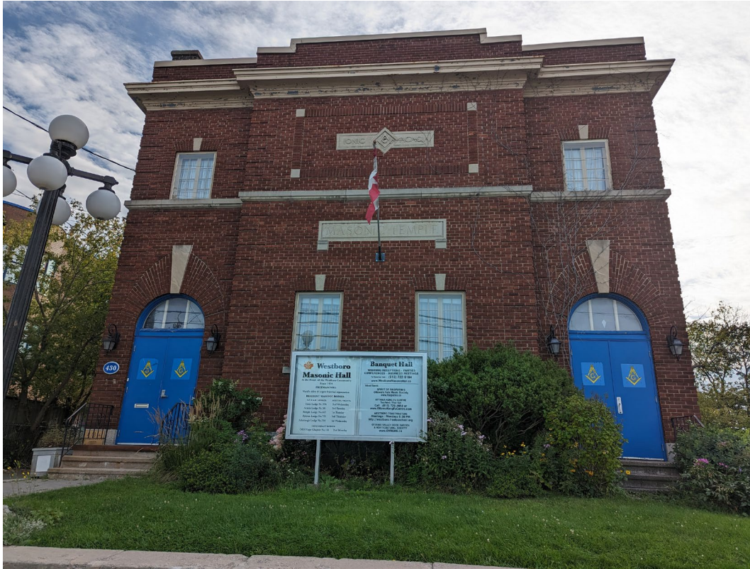
Front façade of 430 Churchill North, looking west. (Source: City of Ottawa, 2023)
