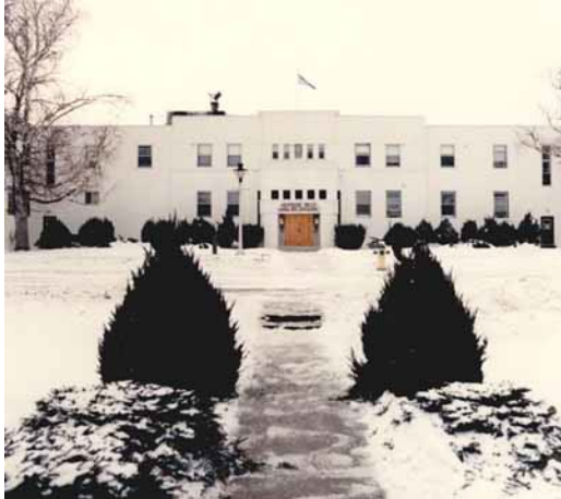
RCAF Officers' Mess at CFB Trenton (Source: Department of National Defence, 1994).
